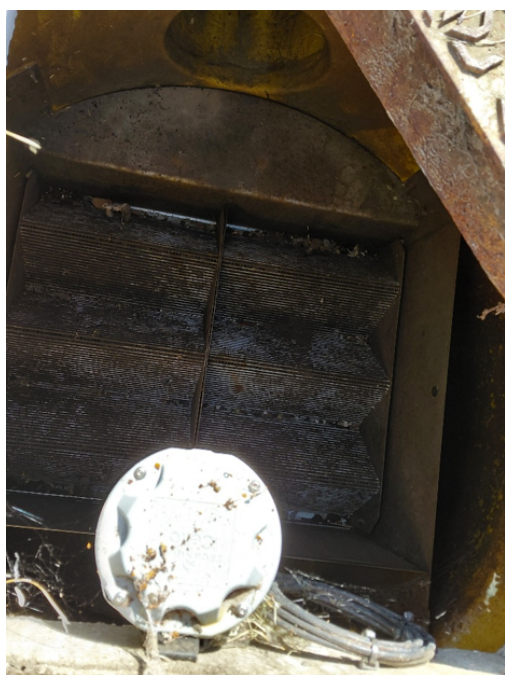
Photograph 1: CSO Monitoring Location with EDM Monitor and Screen
