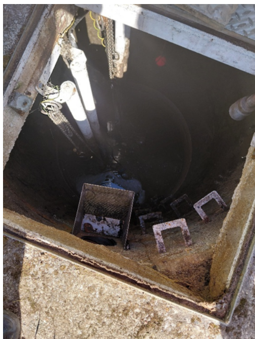
Photograph 1: Overflow Monitoring Location with EDM Monitor and Screen
