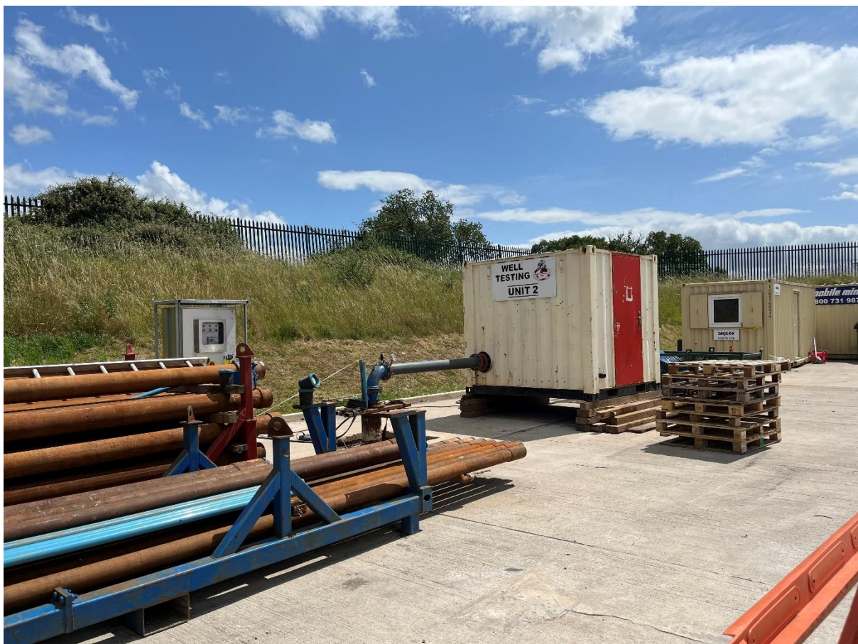
No.2 Borehole undergoing Pump Testing – Summer 2025
