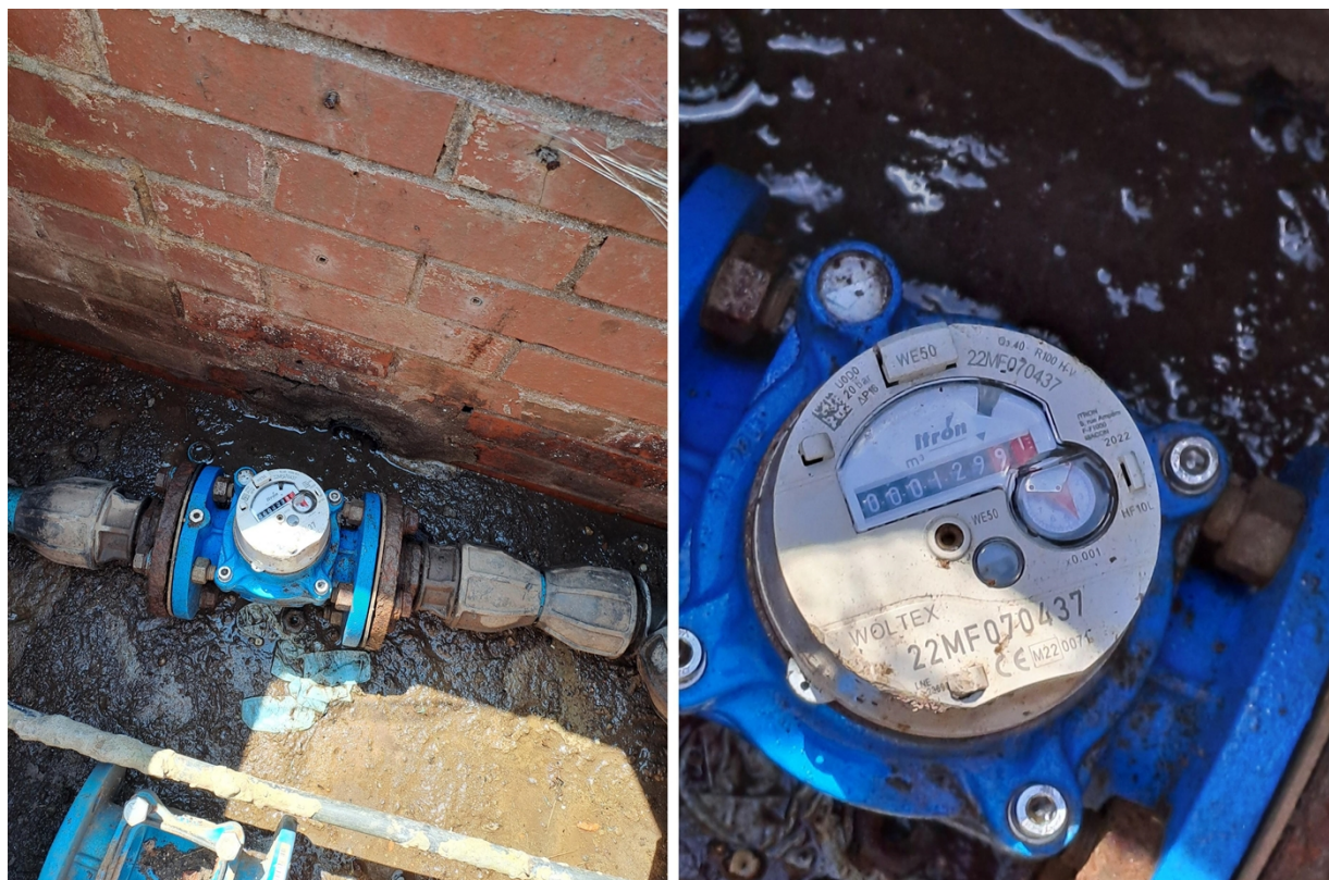
Figure 3 – The water meter as observed during the inspection.
