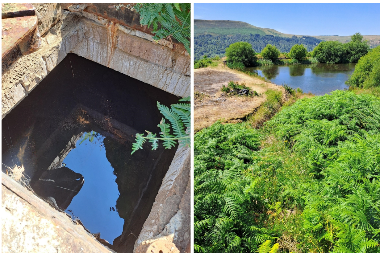
Figure 1 – The abstraction point and overflow to pond as observed during the inspection.
