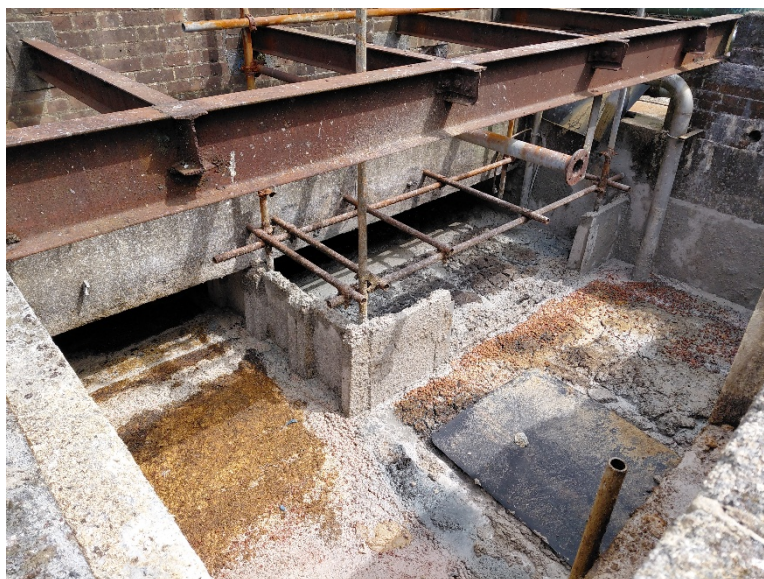
Image 1: View of the Detritus Pit
