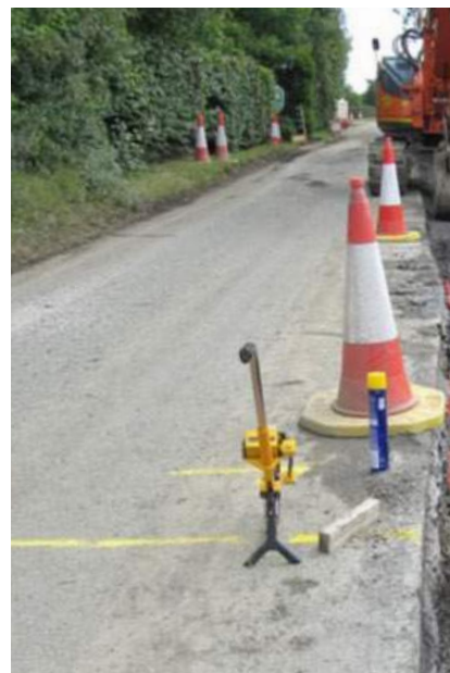
Onshore Cable Installation
