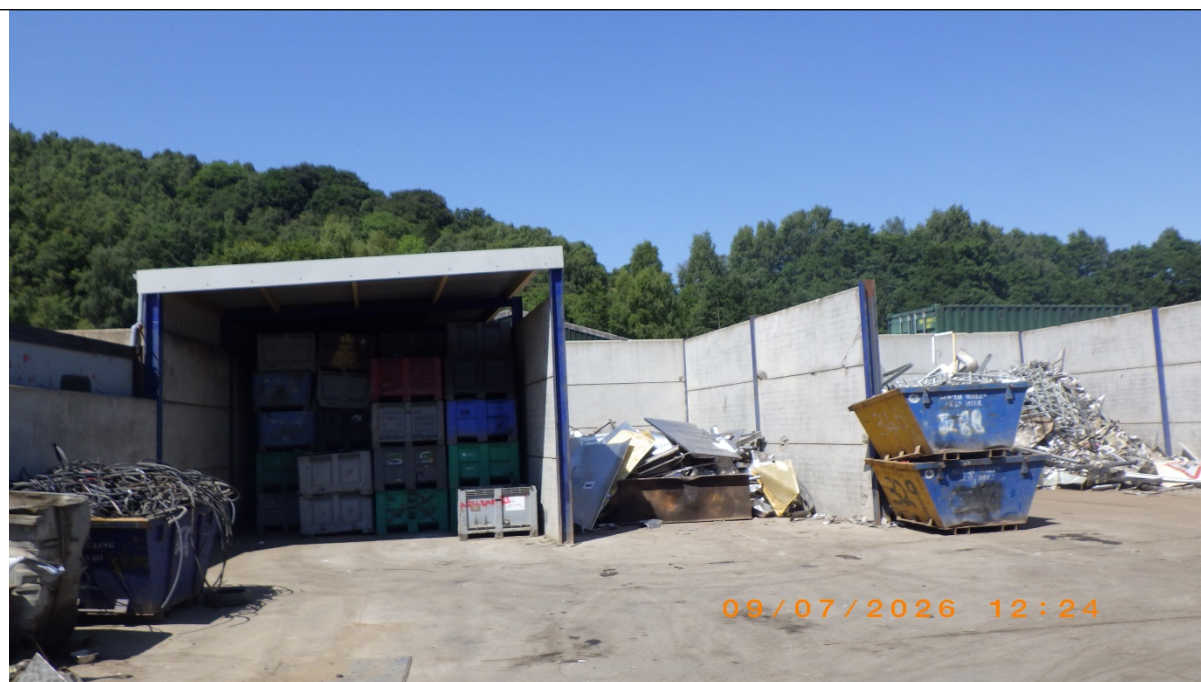
Current batteries storage bay.
