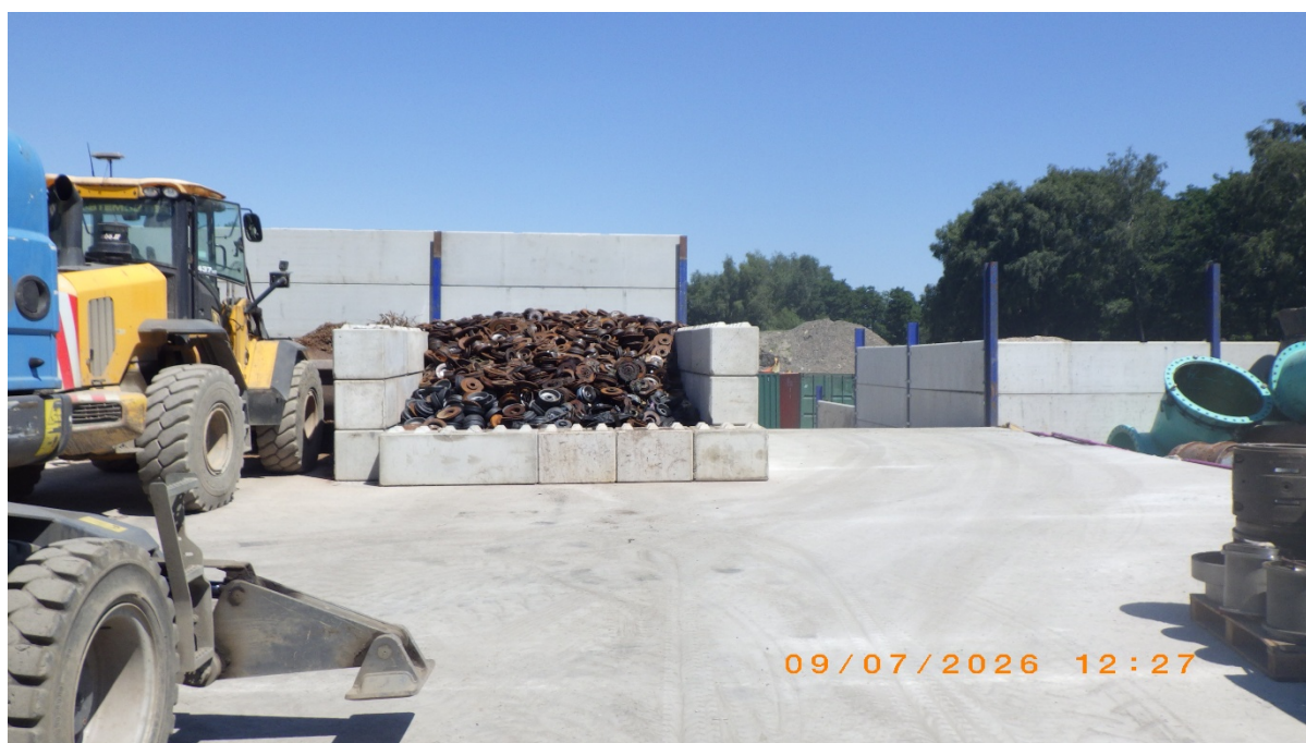
Waste overspilling at the back of the concrete bay
