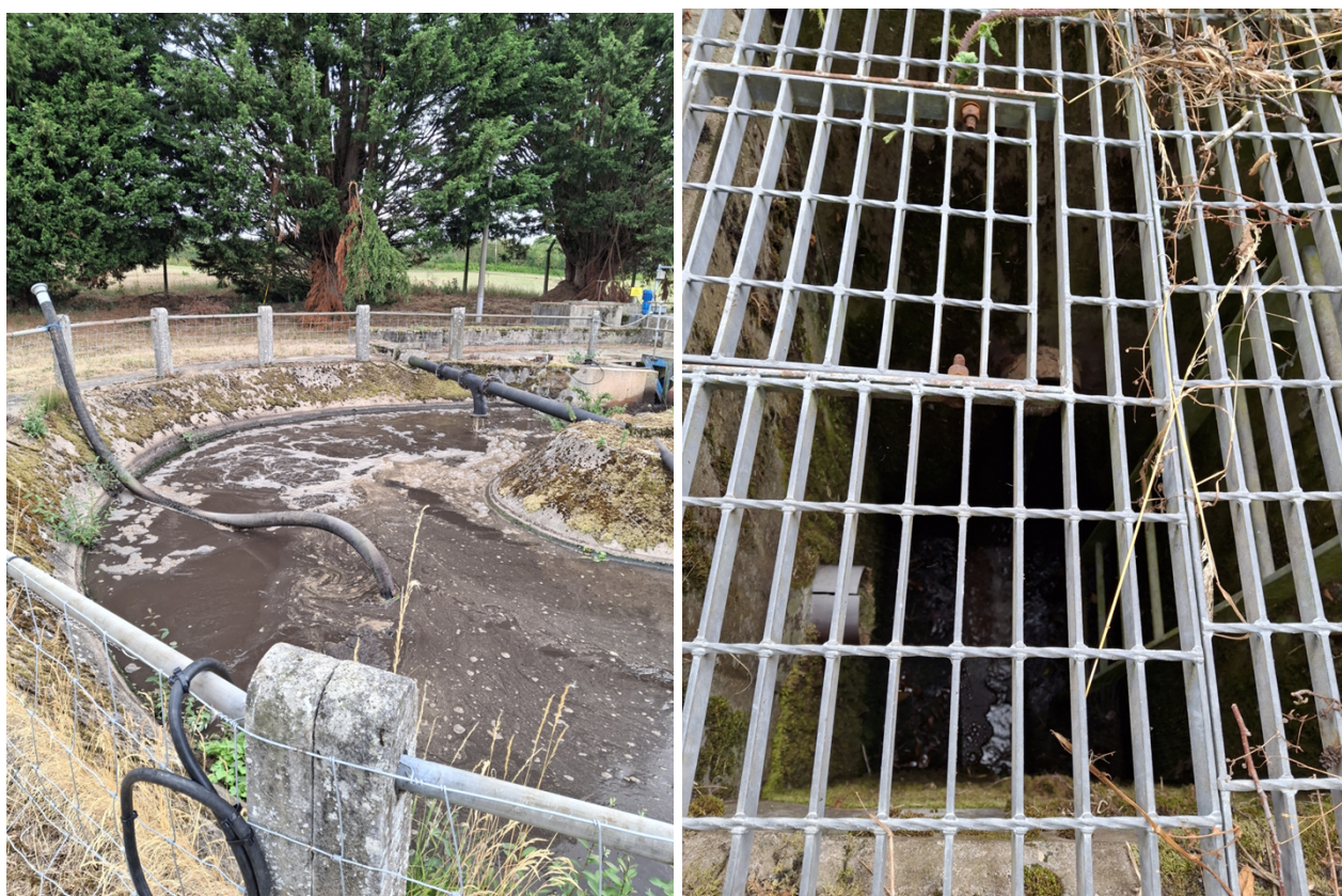
Figure 1. Additional aeration is being provided whilst repairs to the aeration ditch are undertaken (left) and Dwr Cymru / Welsh Water sampling point (right).
