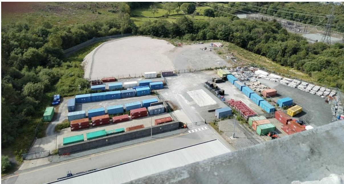
Figure 10 – RCA laydown area (2024)
