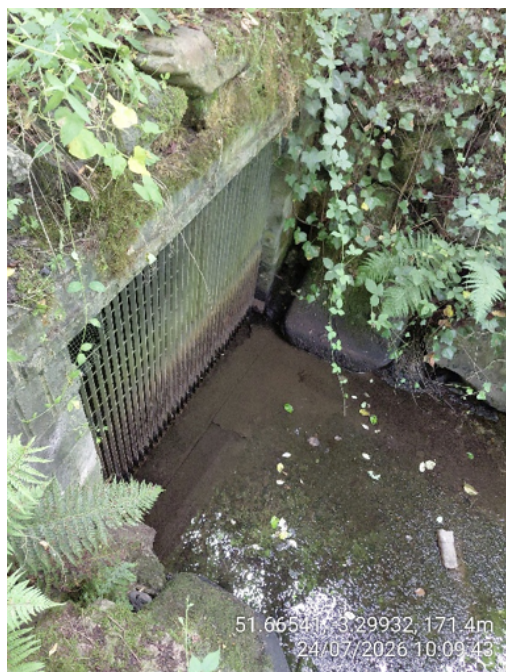
Photograph 1: Outfall from the Turbine House
