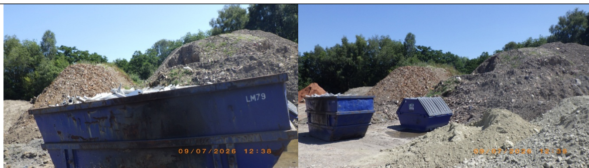
Skip full of metal waste stored next to waste soil
