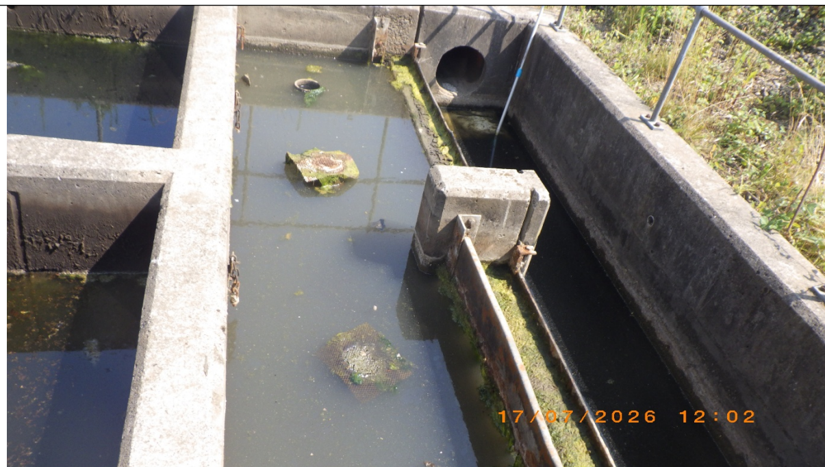
Unblocked outlet pipe
