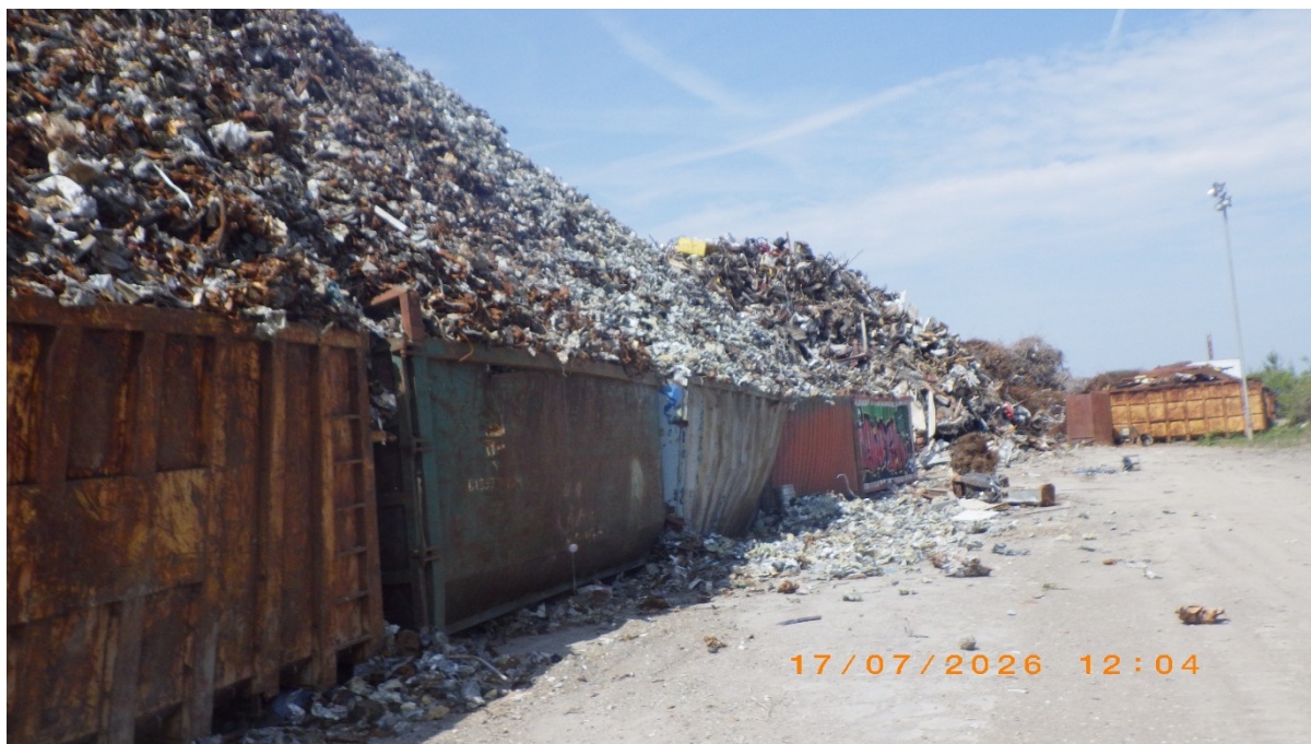
Waste strewn on the ground and overflowing for the storage piles
