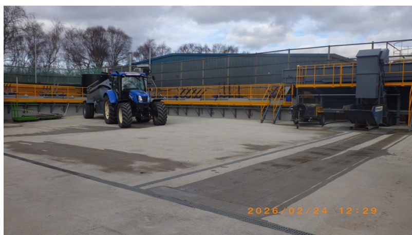
Photograph of new wash bath installed in 'unit 27'
