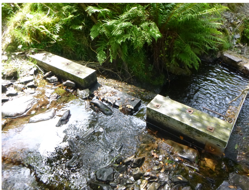
Photograph 3: Stones cleared from HoF notch
