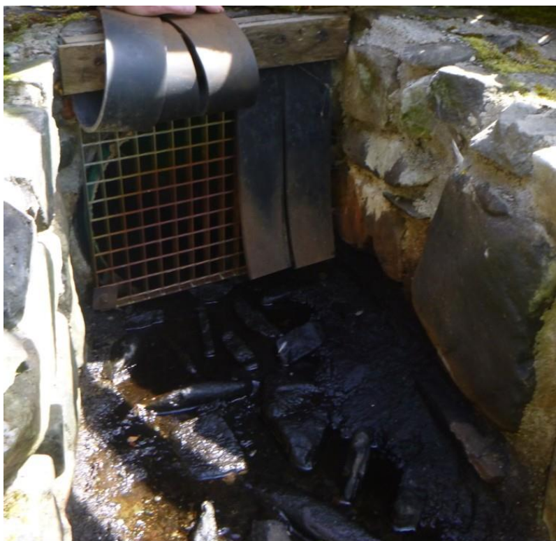
Photograph 4: Discharge outlet pipe
