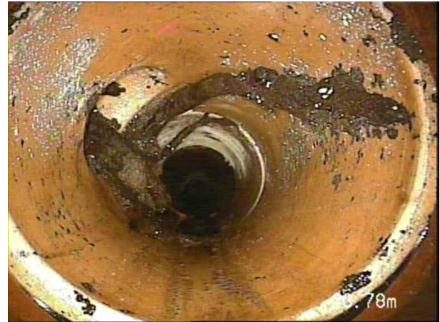
14, 00:04:26, 23.78 m Roots, tap, OUT OF JUNCTION
