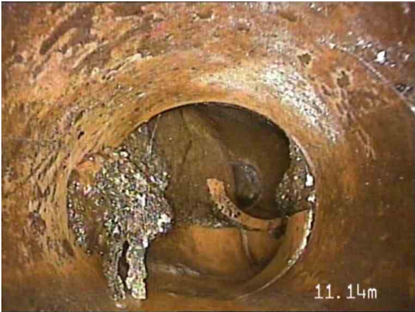
1, 00:01:41, 11.14 m Roots, mass, 15% cross-sectional area loss
