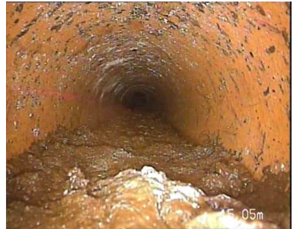
4, 00:02:34, 15.05 m Survey abandoned, UNABLE TO GET PAST SILT
