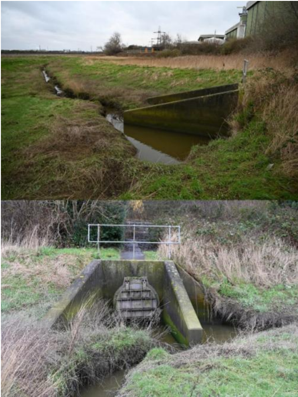
Figure 3: Two perspectives of the Existing Surface Water Outfall (Source: Geomorphological Walkover Survey Report ( EN010166/APP/9.12 ))
