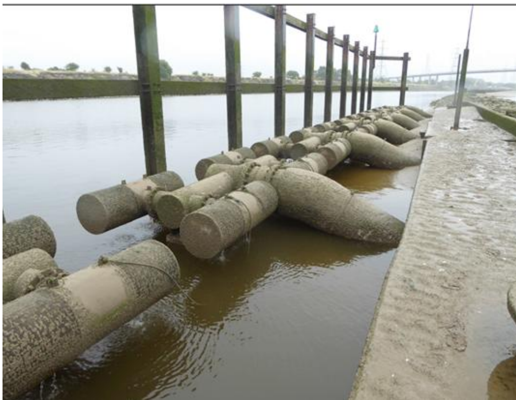
Figure 4: Photograph of existing intake eel screens, intake manifold and steelwork protection 4
