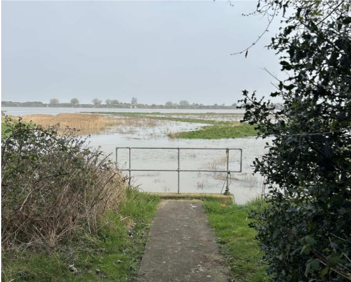
Figure 1: View north towards the Dee Estuary, from existing surface water outfall infrastructure at Connah's Quay power station. Source: Applicant. 11:56am; 20th March 2026.
