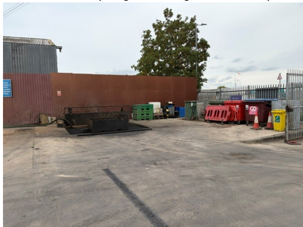
Figure 4 – Concrete floor area near both reception pits. The concrete surface was in excellent condition with no evidence of spillage, staining, residues or pooled liquids.
