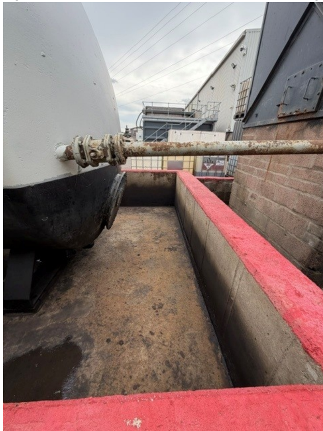
Figure 3 – A section of the concrete bund surrounding reception settlement tank A.
