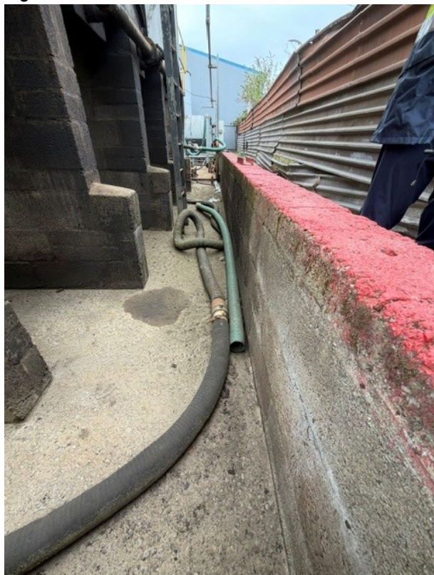
Figure 1 – A section of the unlined breeze block bund wall behind reception tank B.
