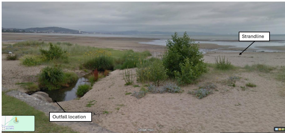
Figure 3 - Existing Outfall at the Proposed Scheme Location in Blackpill, Swansea
