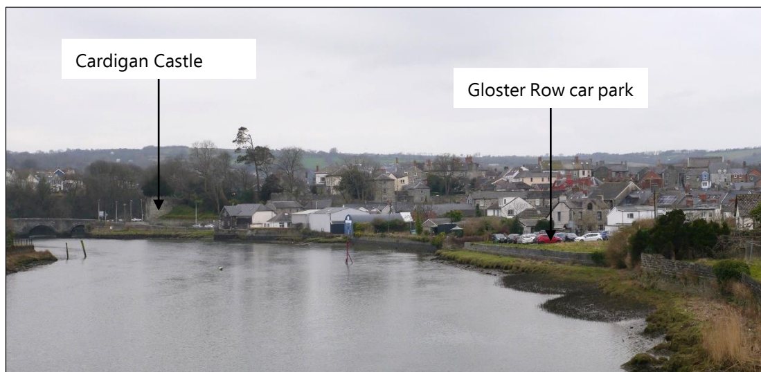
Plate 3-1 – View from Priory Bridge, looking west along the Scheme Area to Cardigan Bridge.
