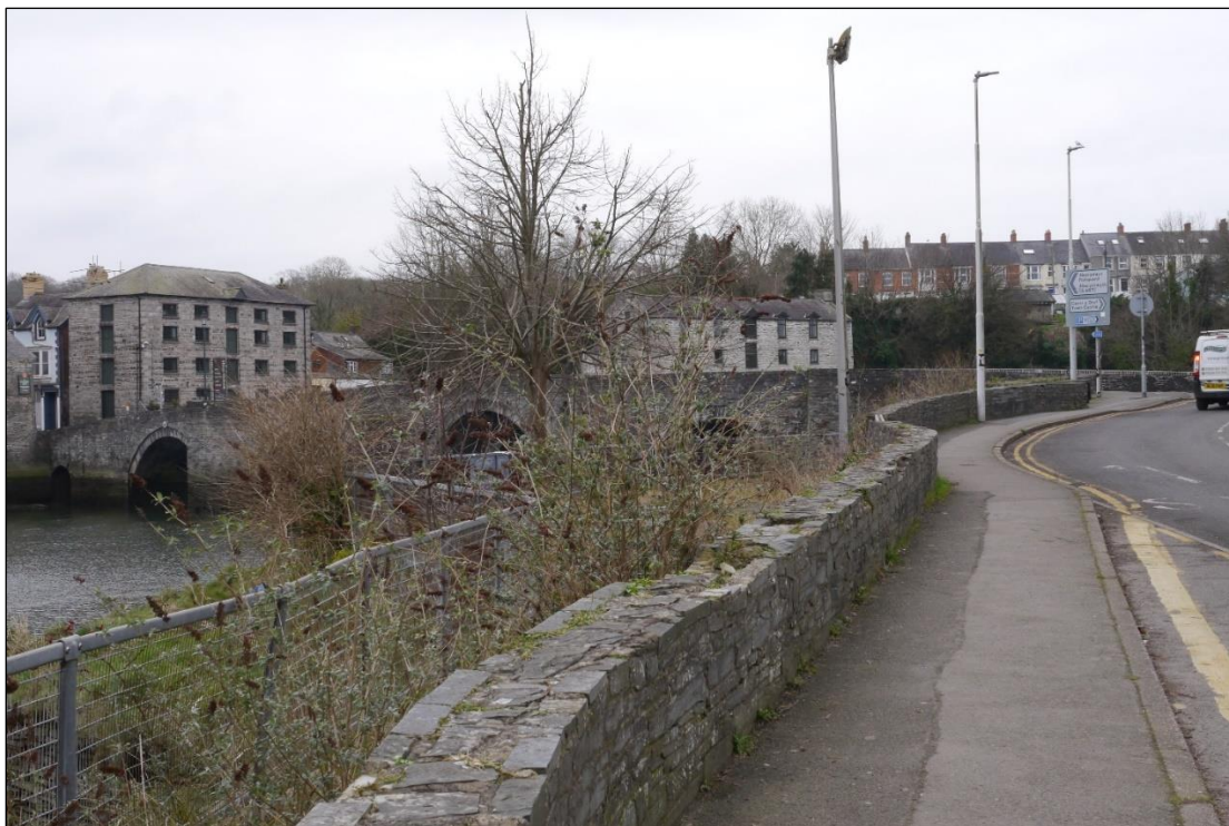
Plate 3-2 – View west along Strand from the bus stop showing the riverside wall, railings and overgrown inaccessible space in between. Cardigan Bridge Scheduled Monument can be seen in the background.
