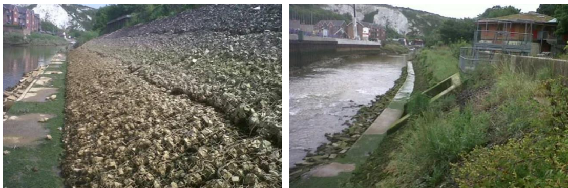
Plate 2-3 – Rock roll mattresses at Railway Lane, Lewes showing development of intertidal habitat over time (images courtesy of Salix)
