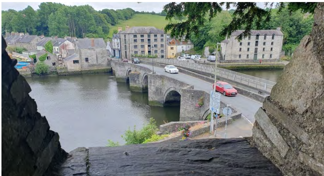
Figure 4 Photograph of the town bridge, looking south across the Afon Teifi, taken during site visit, June 2024
