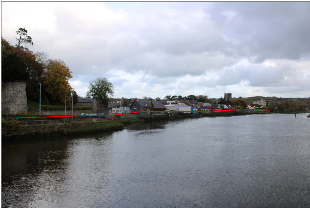
Photo 4: View of the Scheme from midway along Cardigan Bridge. Indicative line of new riverside wall in red (for approximate reference only, not included to scale).
