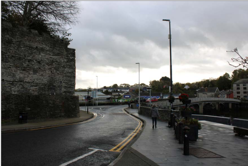
Photo 23: View from the southern end of Bridge Street with Cardigan Castle on the left and Cardigan Bridge on the right.
