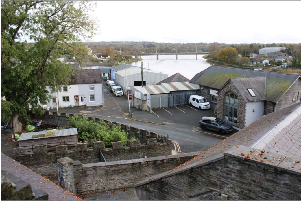
Photo 11: View from Cardigan Castle walls, overlooking the old stables and towards the Scheme. Indicative line of new riverside wall in red (for approximate reference only, not included to scale).
