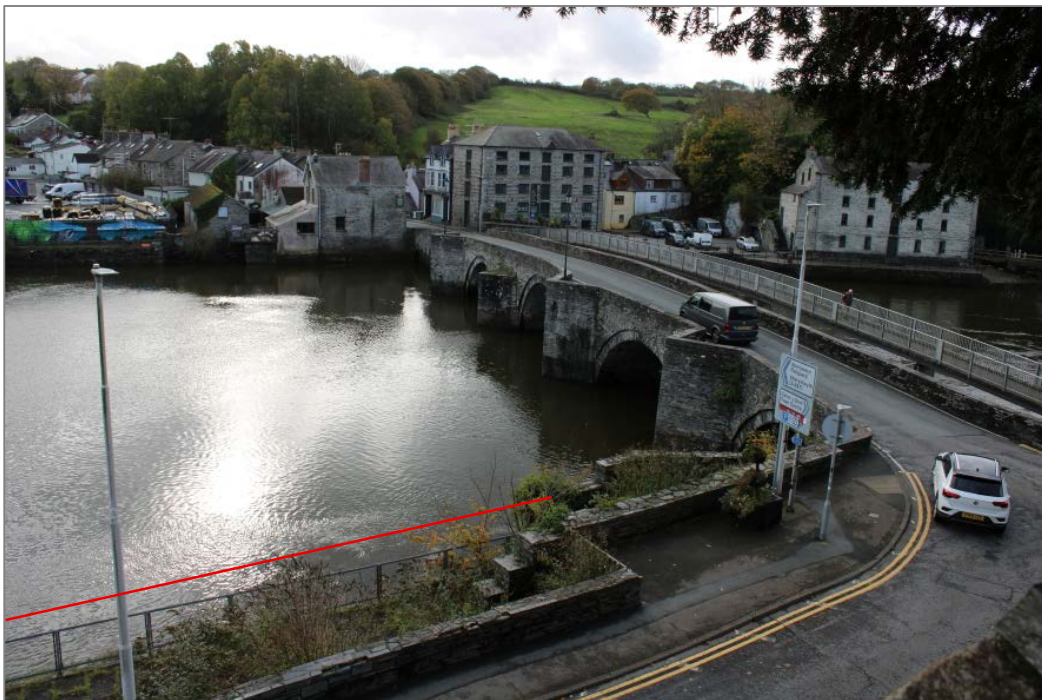
Photo 8: View from Cardigan Castle walls overlooking Cardigan Bridge. Indicative line of new riverside wall in red (for approximate reference only, not included to scale).
