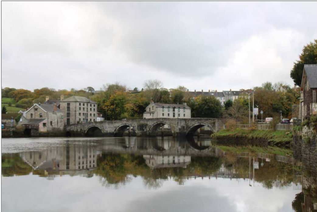
Photo 1: View of Cardigan Bridge from the current riverside wall, with the Castle Inn on the left and warehouses behind, all listed buildings.
