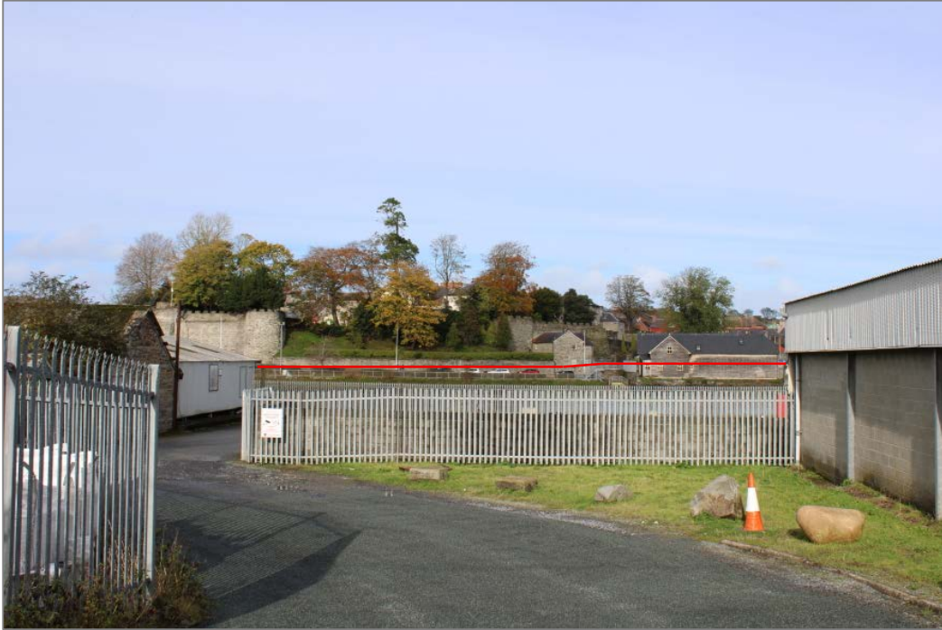
Photo 17: View of the Scheme from Station Road on the south side of the river. Indicative line of new riverside wall in red (for approximate reference only, not included to scale).
