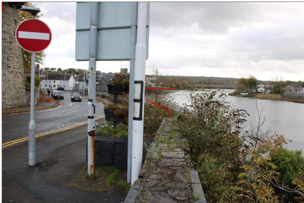
Photo 2: View of the Scheme area from the north side of Cardigan Bridge. Indicative line of new riverside wall in red (for approximate reference only, not included to scale).
