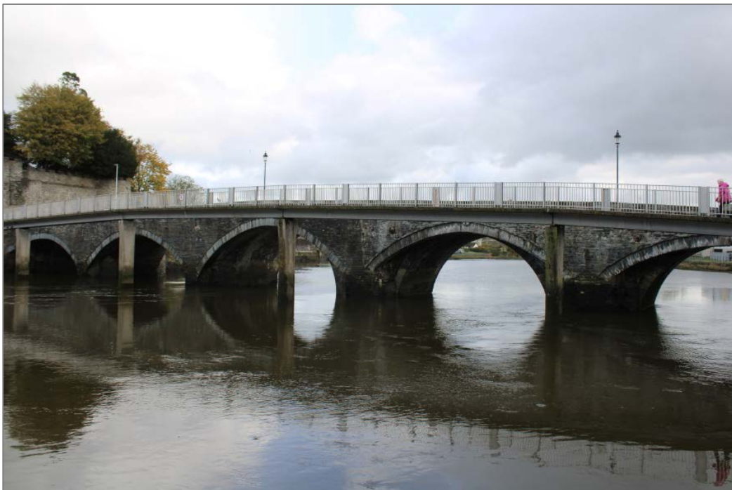
Photo 24: View towards the Scheme from the southern riverside to the west of Cardigan Bridge. The Scheme would be intermittently visible through the arches.
