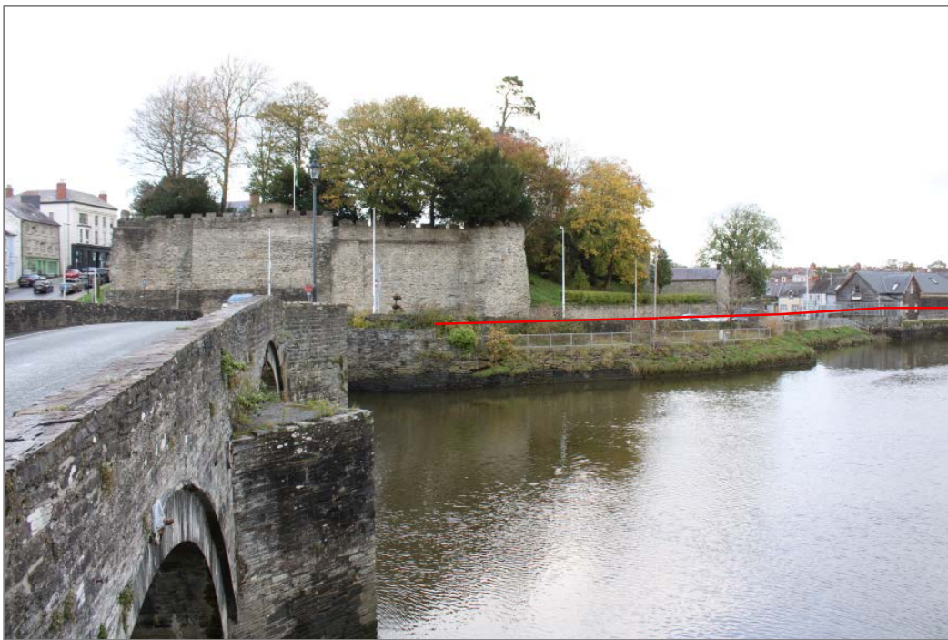
Photo 6: View from the south side of Cardigan Bridge (adjacent to the Castle Inn), also showing Cardigan Castle. Indicative line of new riverside wall in red (for approximate reference only, not included to scale).
