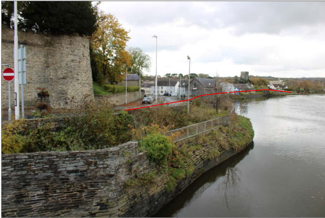
Photo 3: View of the Scheme from the northern end of Cardigan Bridge. Indicative line of new riverside wall in red (for approximate reference only, not included to scale).
