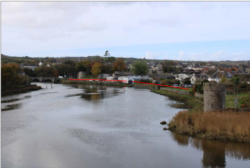
Photo 16: View of the Scheme from Priory Bridge. Indicative line of new riverside wall in red (for approximate reference only, not included to scale).
