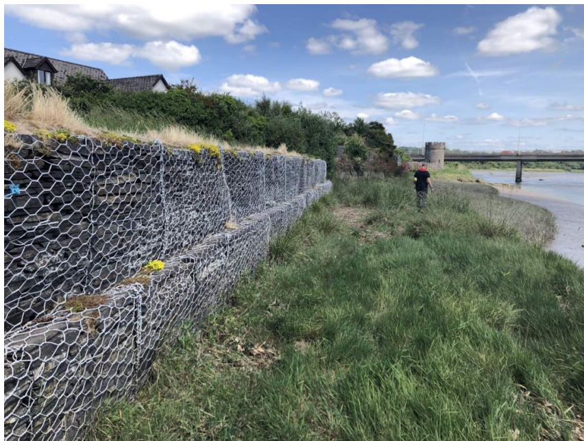
Figure a-2 - Gabion defences, facing upstream with the grounds of St Mary's Church in the background (ID: 66).
