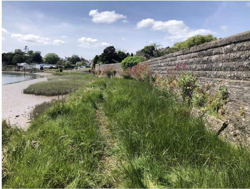
Figure a-1 - Flood defence wall, surrounding the grounds of St Mary's Church, facing downstream (ID: 90).
