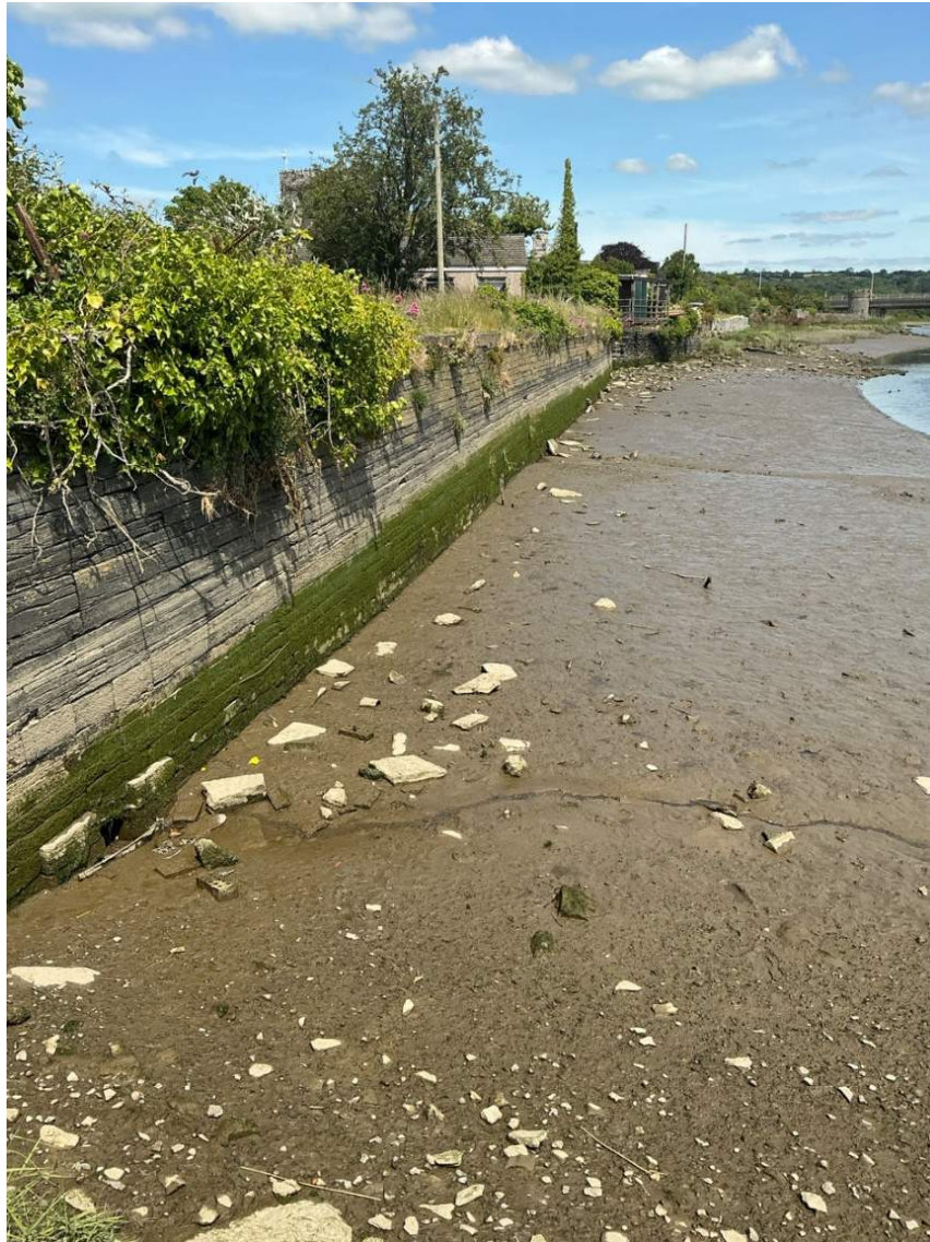
Figure a-3 – Flood defence wall upstream of the activity centre slipway (ID: 142).
