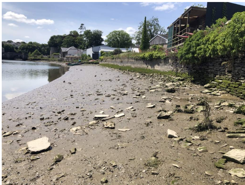
Figure b-1 – Upstream intertidal habitat that will be lost by the engineered riverbank realignment, facing downstream (ID: 62).
