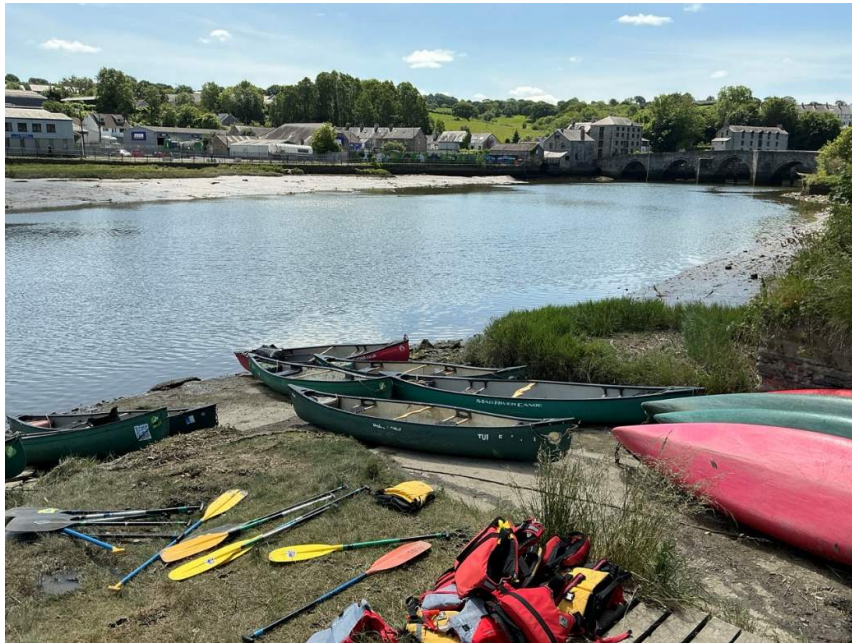
Figure d-2 – Downstream slipway, used for recreational boating activities by the adventure centre (ID: 36).
