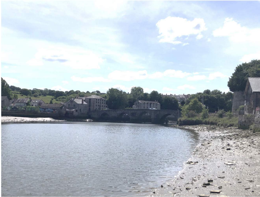
Figure e 5 – Cardigan Bridge, viewed from the right bank facing downstream (ID: 127).
