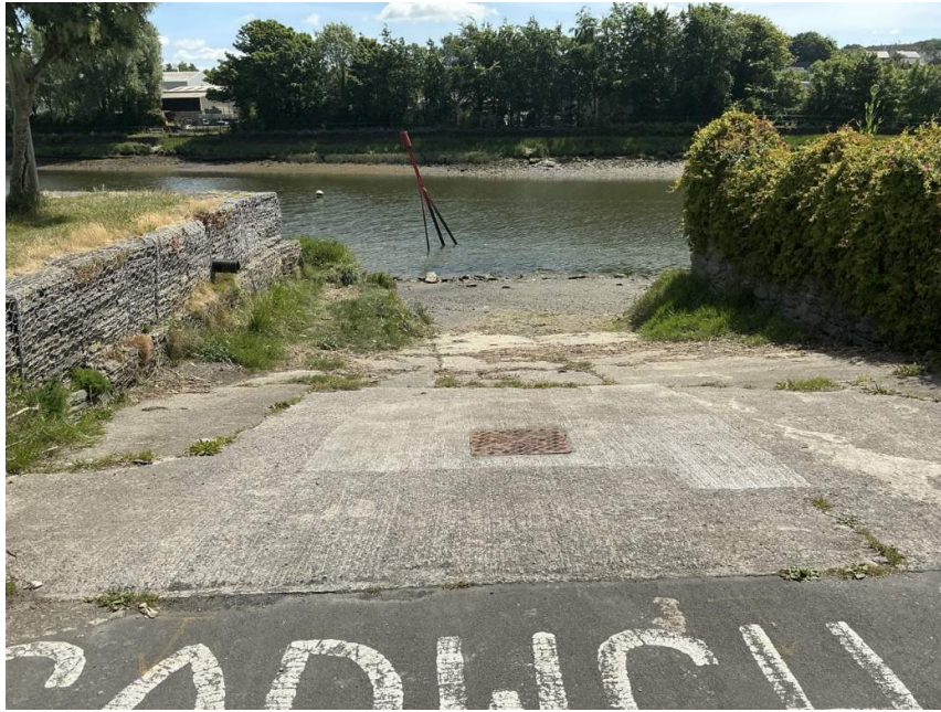
Figure d-1 – Upstream public slipway at Gloster Row Car Park (ID: 73).
