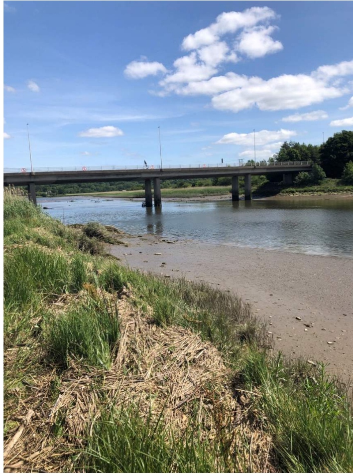
Figure e-4 – Pont Y Priordy (A487), viewed from the right bank facing upstream (ID: 88).
