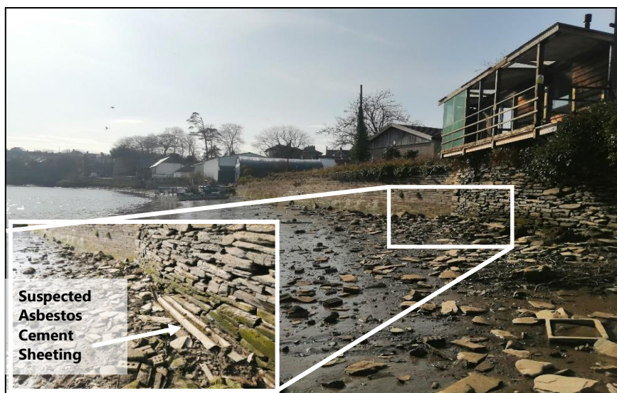
Figure 4-1 – Possible asbestos cement sheeting identified on foreshore in 2022.
