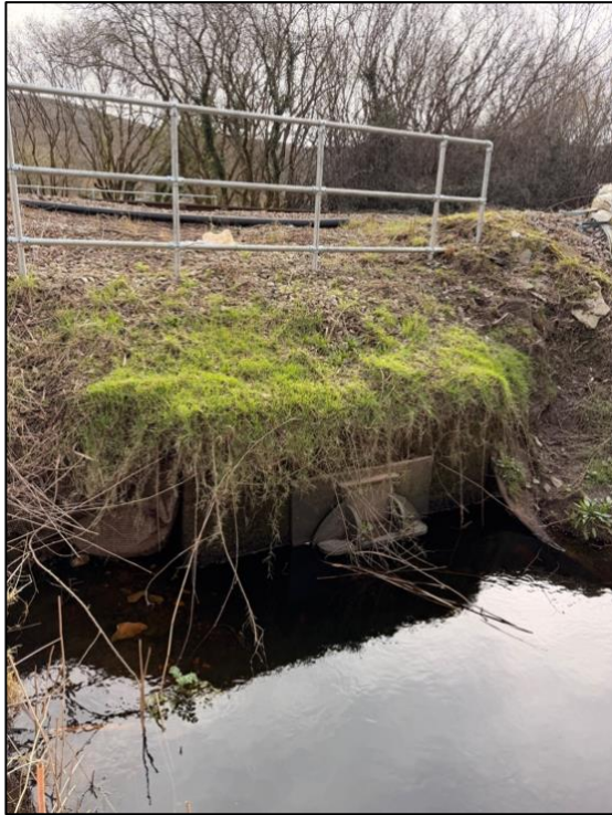
Figure 6: Tidal flap and headwall to be replaced.
