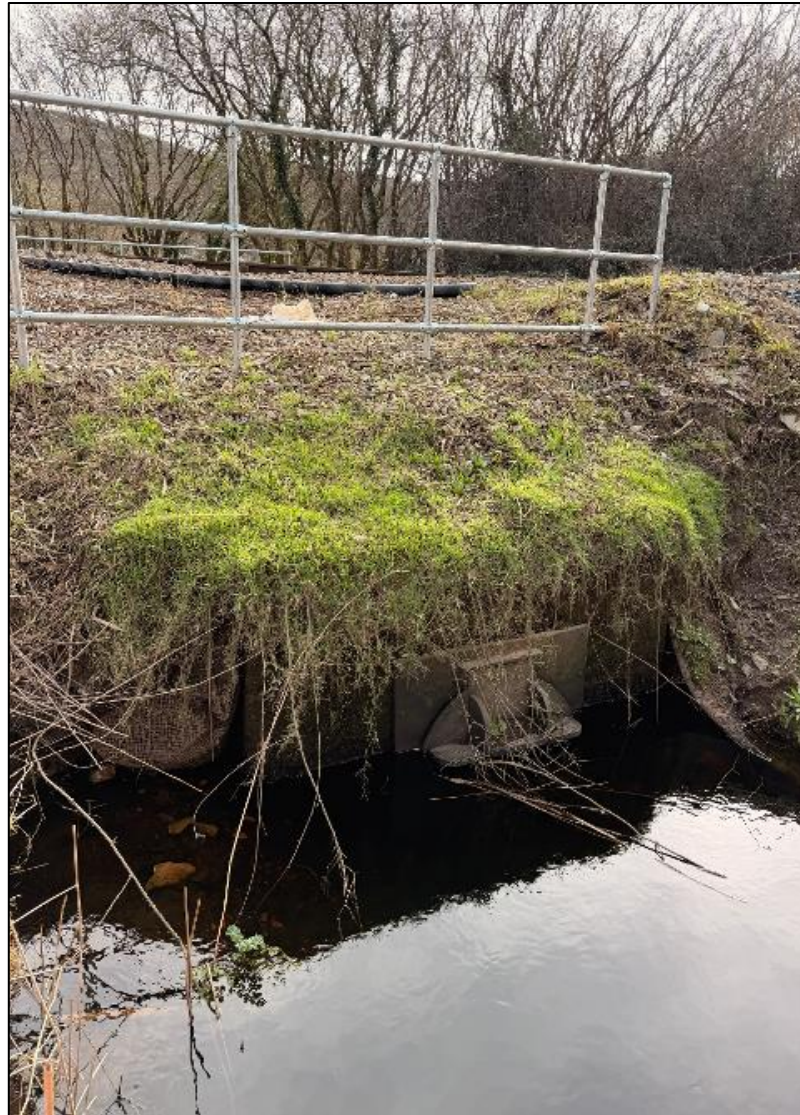
Figure 1: Dovey Junction Tidal Flap.
