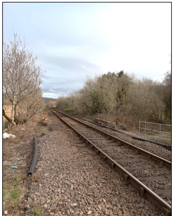
Figure 7: Surrounding Rail Corridor.
