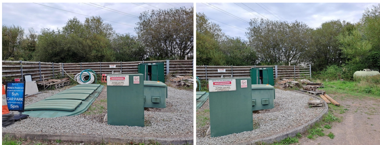
Figure 1 – The site compound as observed during the inspection.
