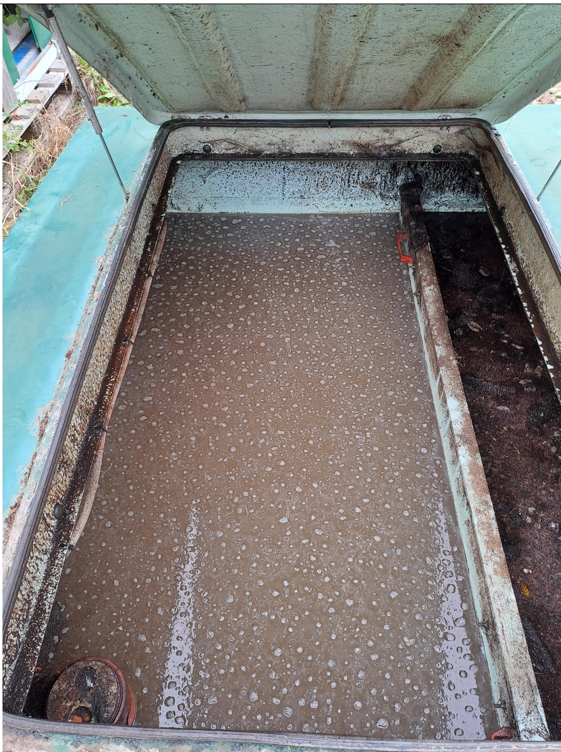
Figure 4 – The secondary treatment tank as observed during the inspection.
