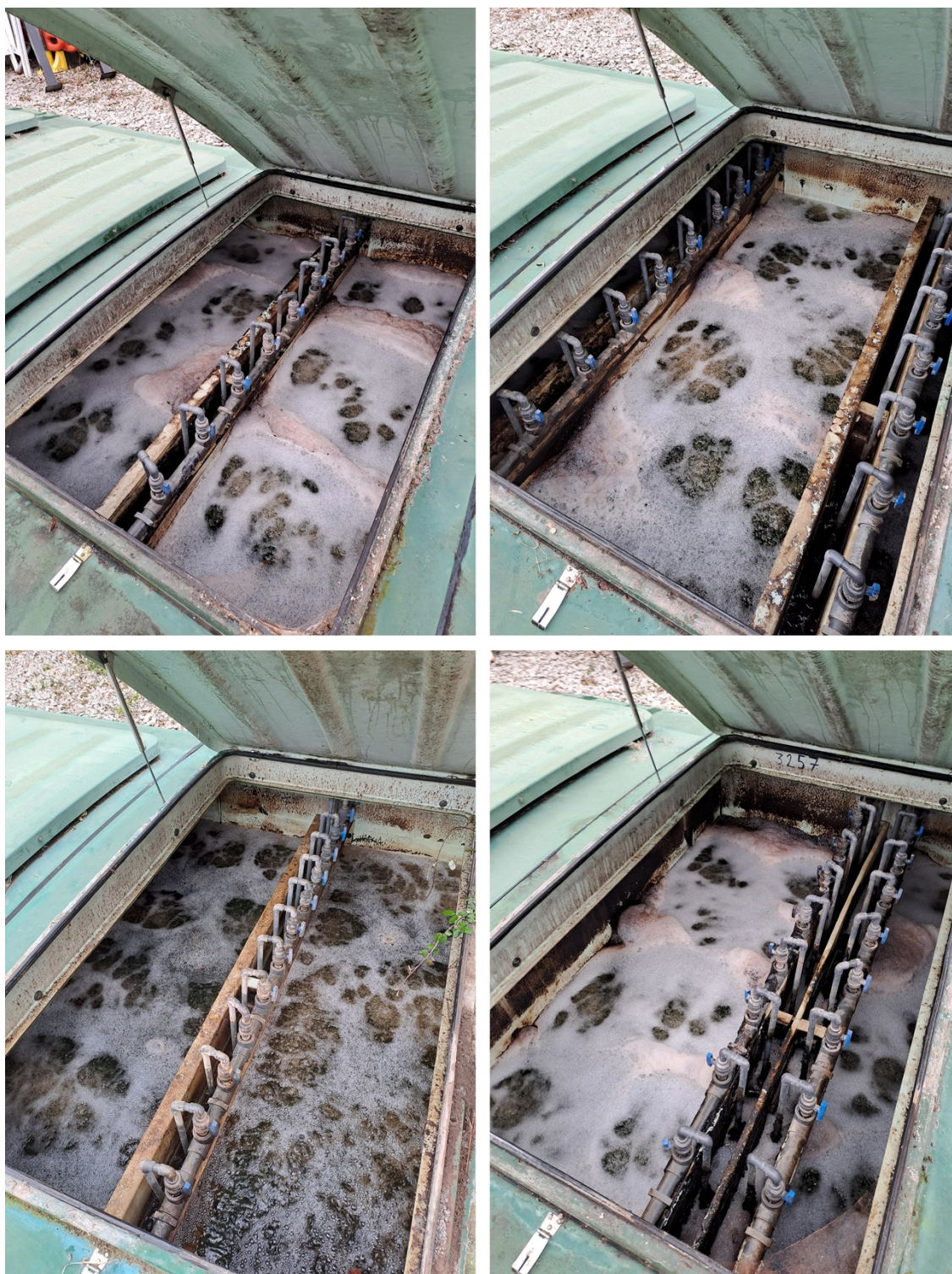
Figure 5 – The aeration chambers as observed at the time of the inspection.
