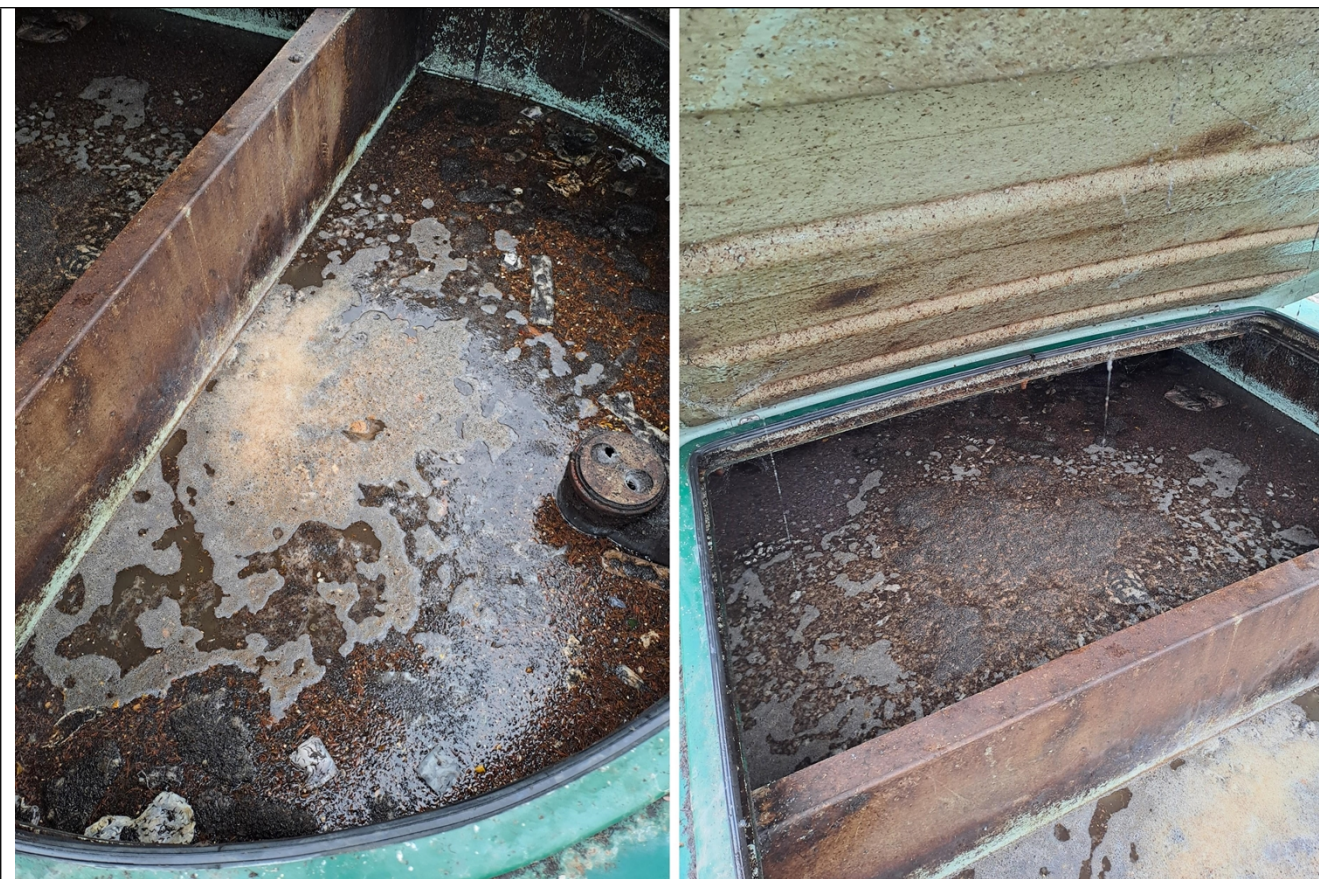
Figure 3 – The primary settlement tank as observed during the inspection.
