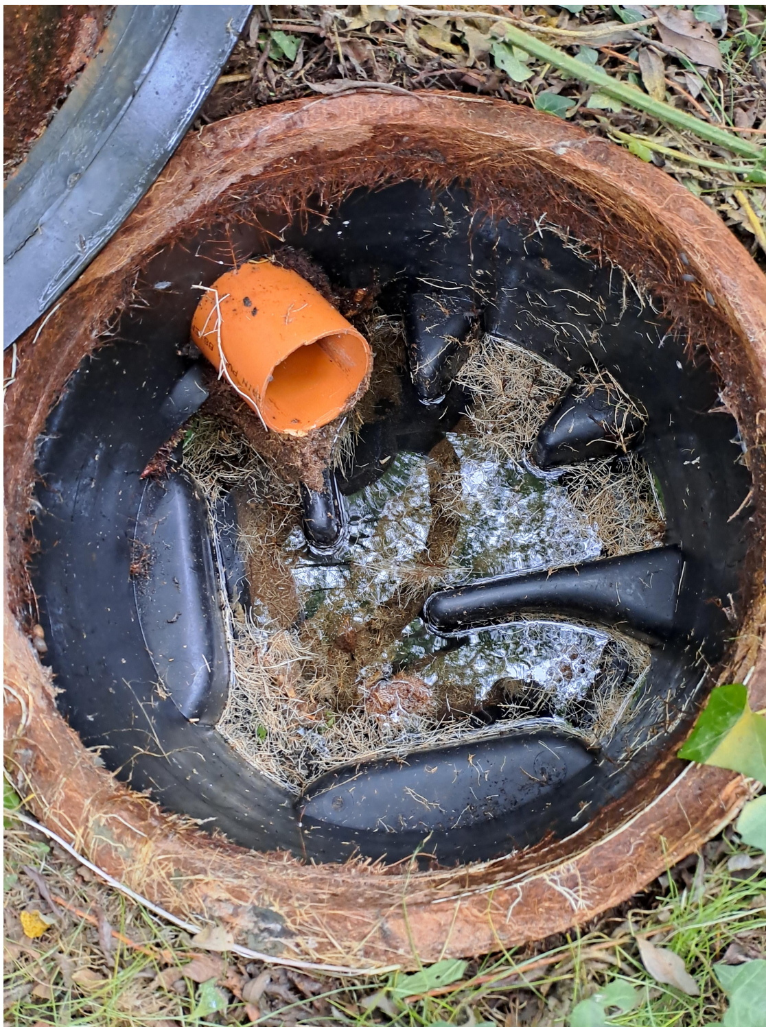
Figure 7 – The sample point as observed during the inspection.
