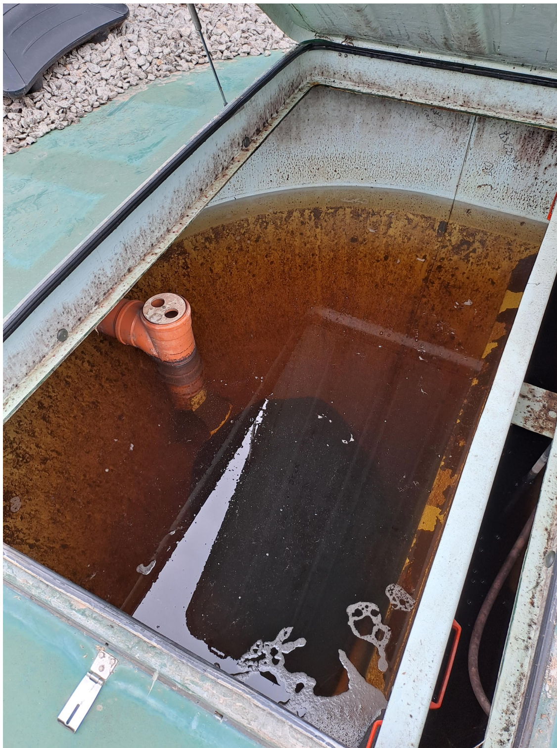
Figure 6 – The final effluent chamber as observed during the inspection.
