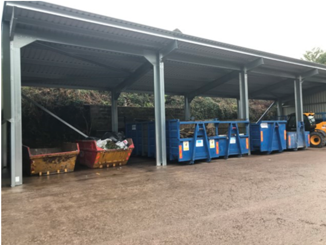
Photo – New site building
