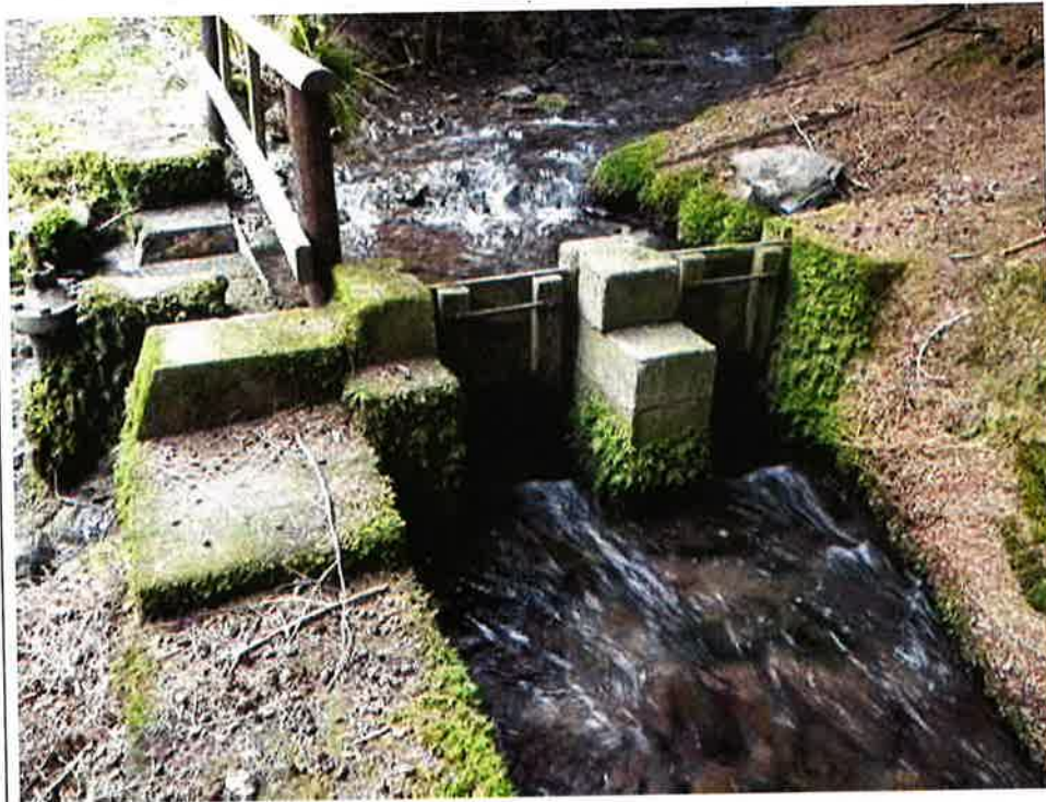
Residual flow notch blocked by board. No hands off flow notch. This notch should pass 7 litres per second plus 50% of the flow in the watercourse downstream.
