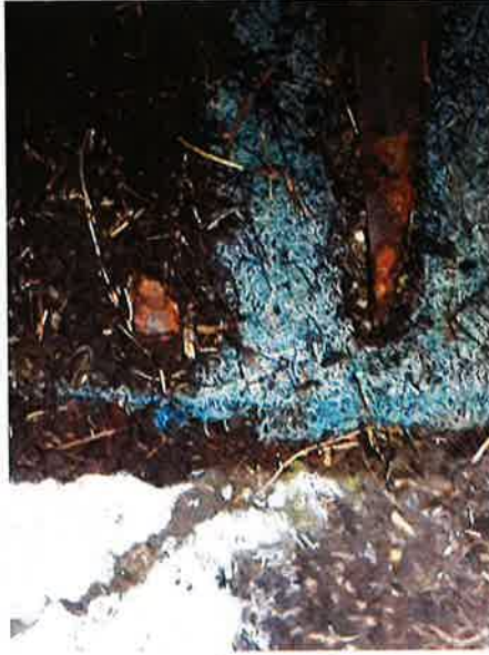
Filter mat in Off-take Chamber (Photo 6)
