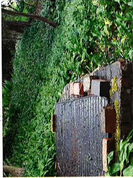
Domestic supply Off-take Chamber (Photo 5)
