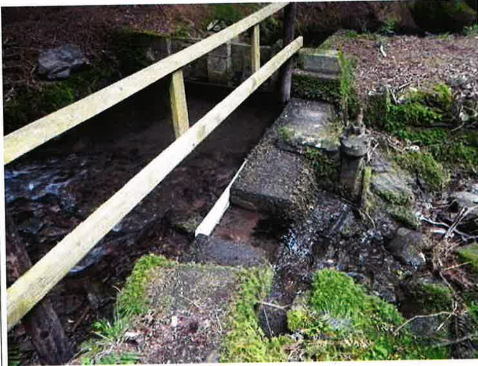
Residual flow notch blocked by board. No hands off flow notch. This notch should pass 7 litres per second plus 50% of the flow in the watercourse downstream.
