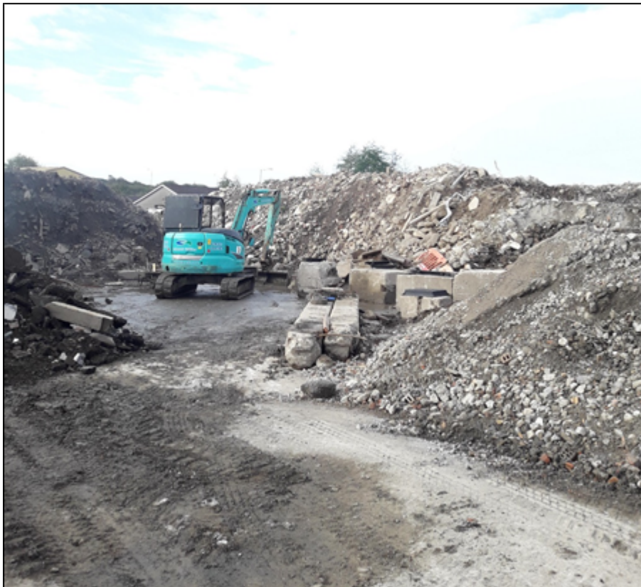
Image 1 – showing mixed concrete piles stored on impermeable infrastructure
