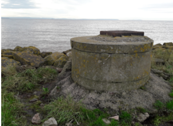
Photo 5: Manhole near Discharge point
