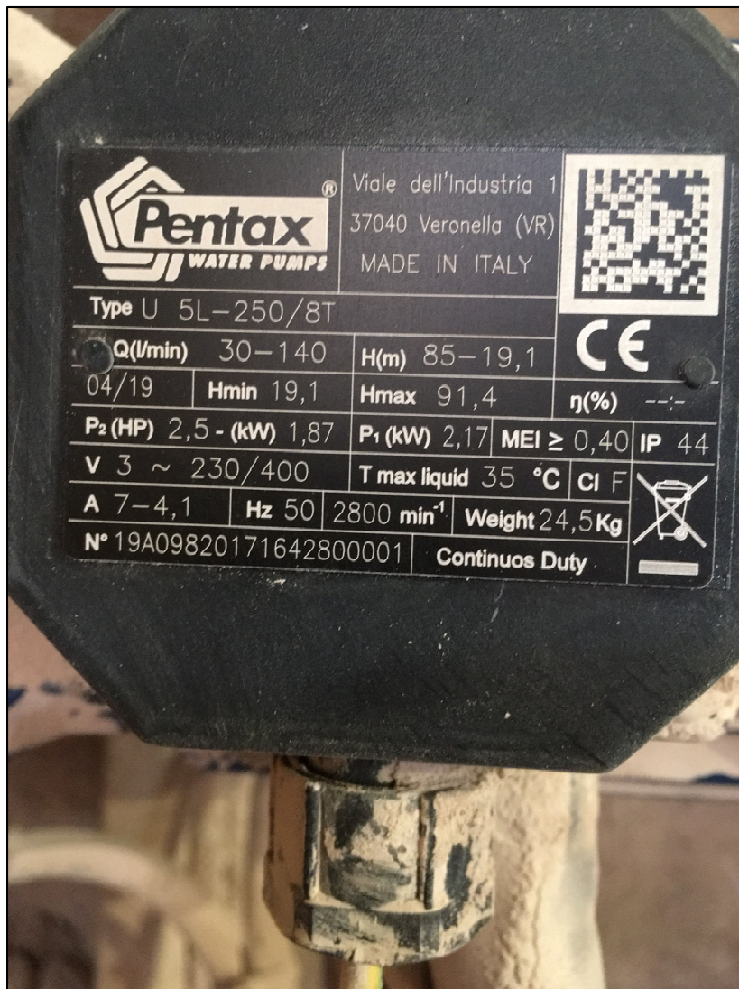
Photo 3 – Nameplate of Pentax ULTRA 5L-250/8T pump used for dust suppression at plant with accompanying pump performance curve (curve 8) (12/07/19 12:17)
