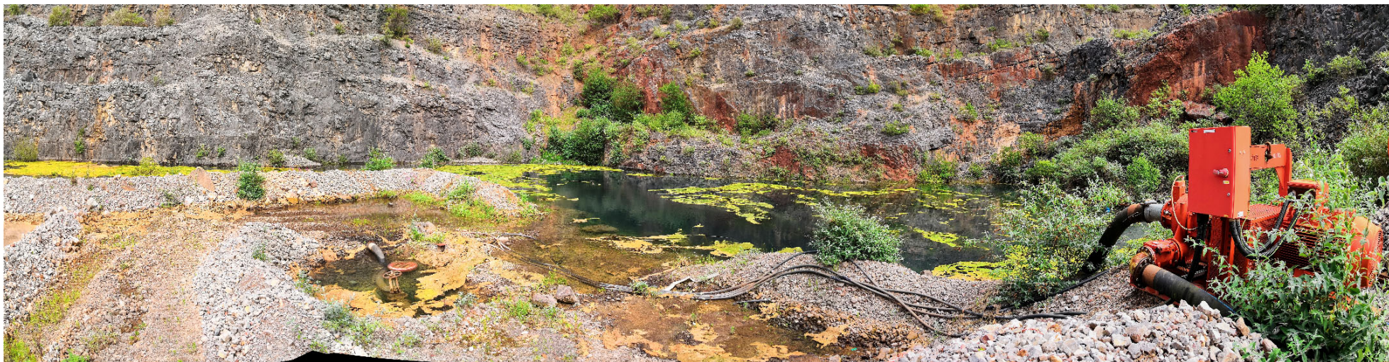
Photo 1 – Panorama of Forest Wood Quarry sump (A1) with dewatering facilitated by a 10" Godwin HL260M pump (26/06/19 13:09)
