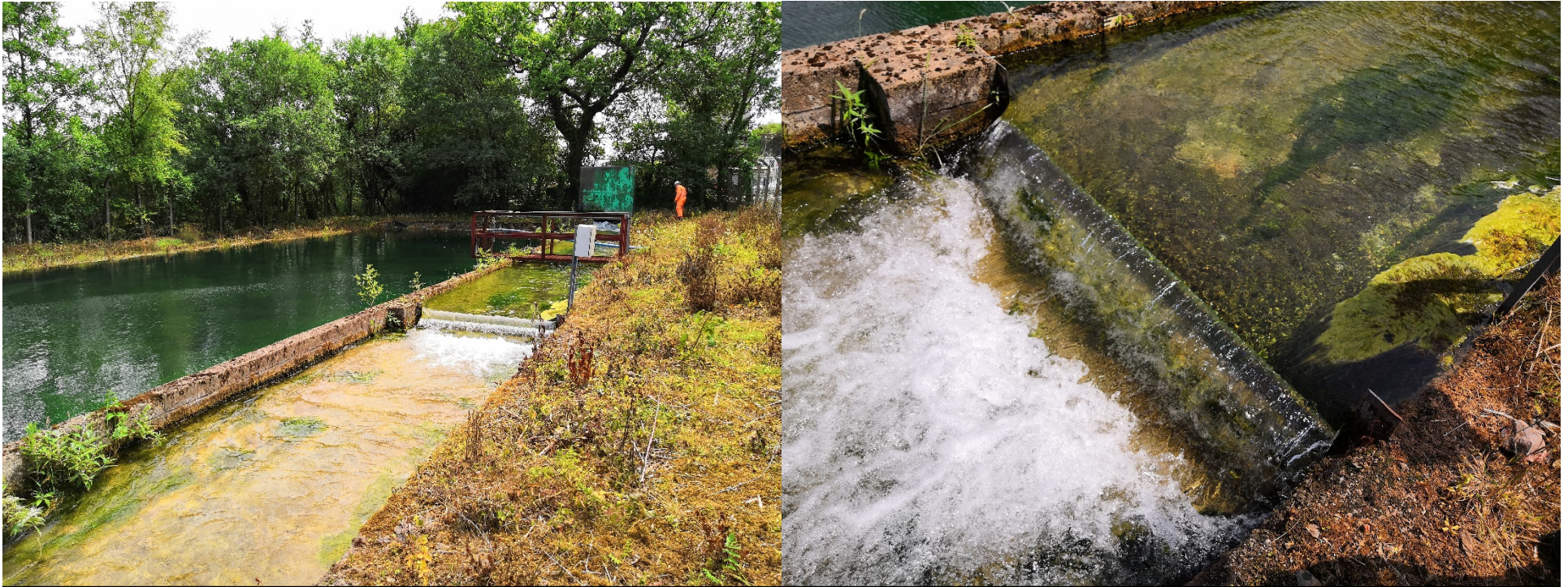
Photos 4 and 5 – Water discharging from quarry sump (A1) passing a weir before entering the settlement lagoon (A2). The grey box next to the weir houses the logger which is used to record the height of water above the weir in 15 minute intervals (26/06/19 13:50)
