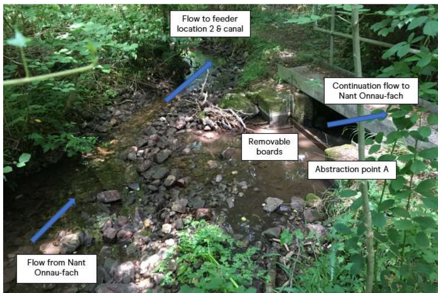
Photo 4: Removable boards location 2, looking upstream. Flow diverted to canal 25/07/18
