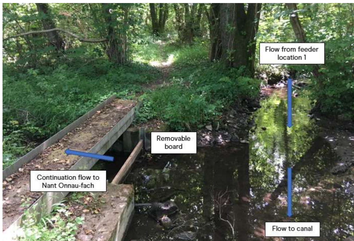
Photo 4: Removable boards location 2, looking upstream. Flow diverted to canal 25/07/18
