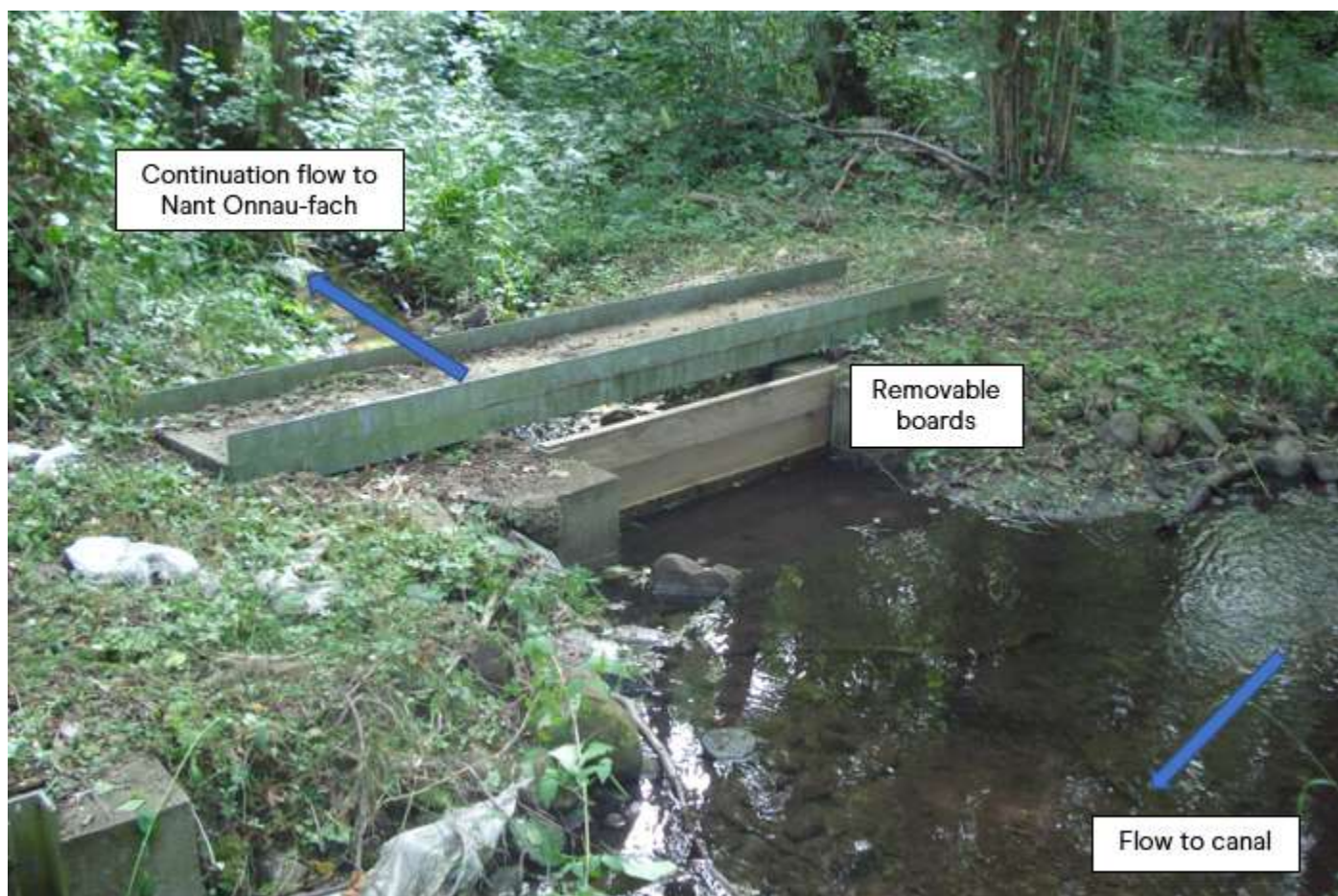
Photo 6: Removable board locations 2 and 3. Flow diverted to canal 17/08/11
