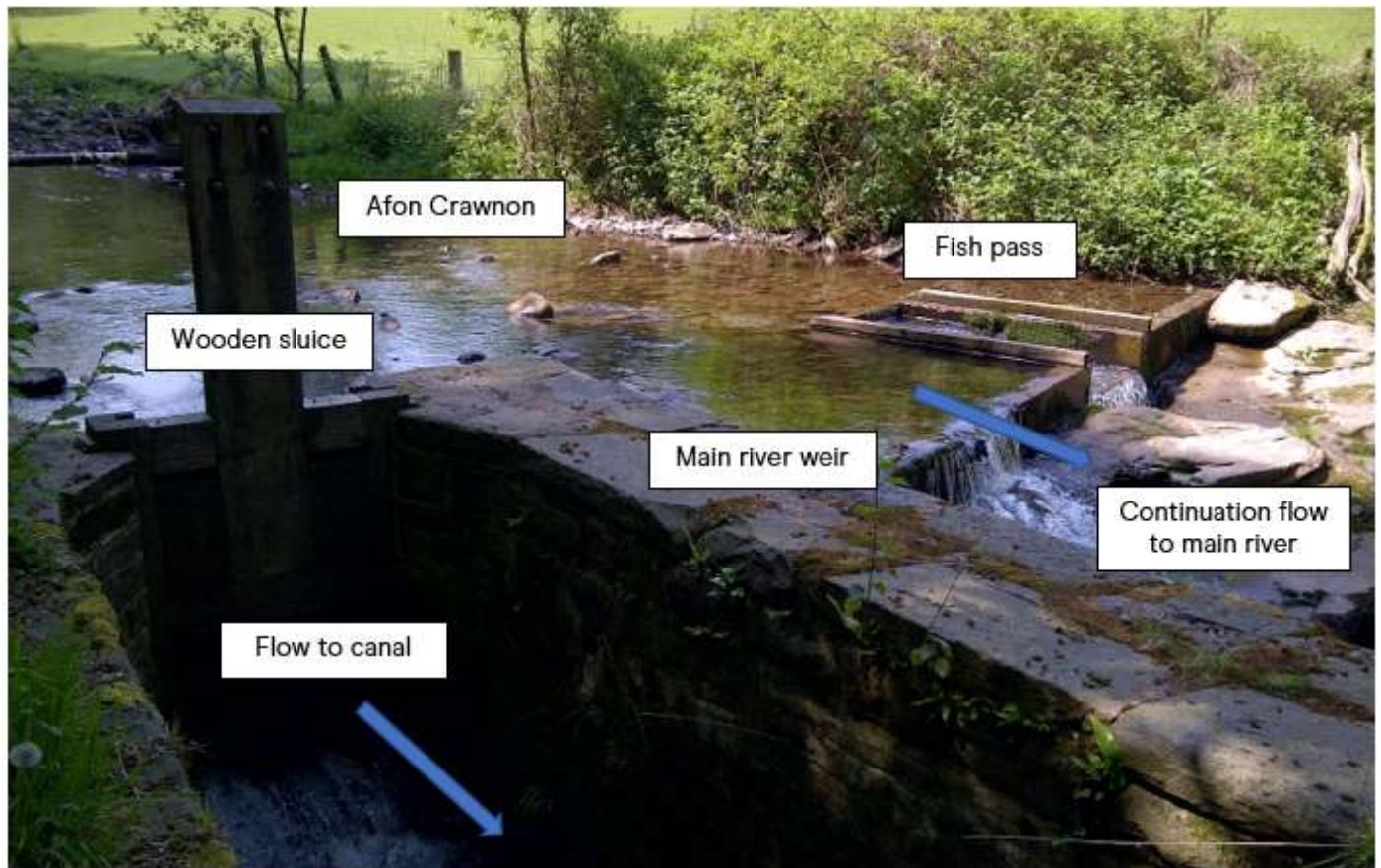
Photograph 2: Wooden sluice 25.05.12
