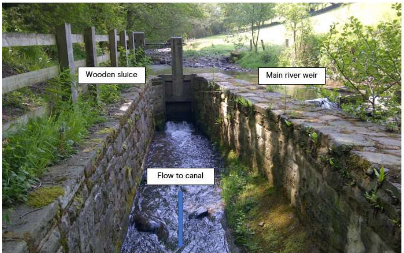
Photograph 3: Abstraction structures looking upstream – sluice and main river weir 25.05.12
