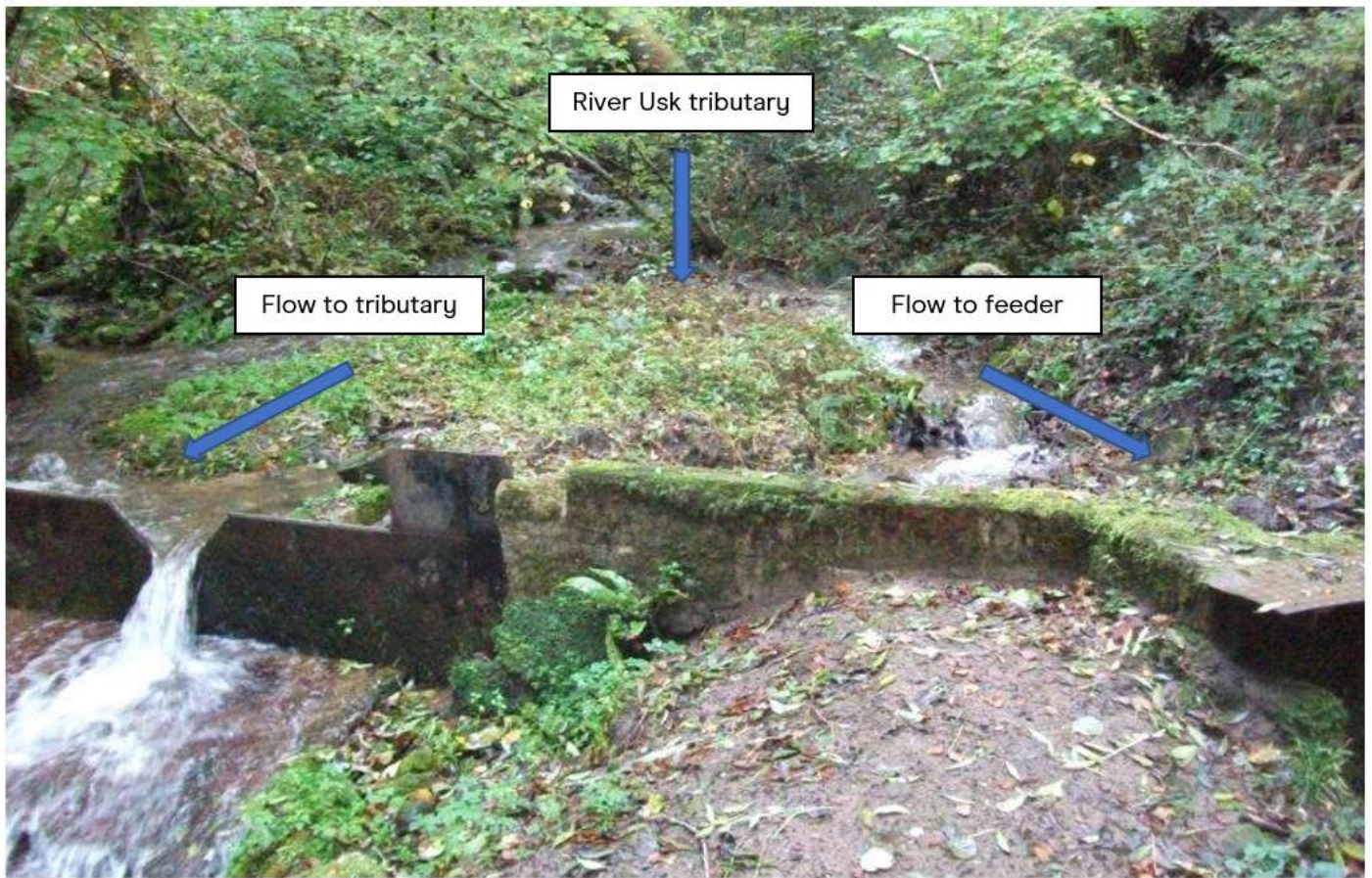
Photo 2: Sluice to feeder channel, looking downstream
