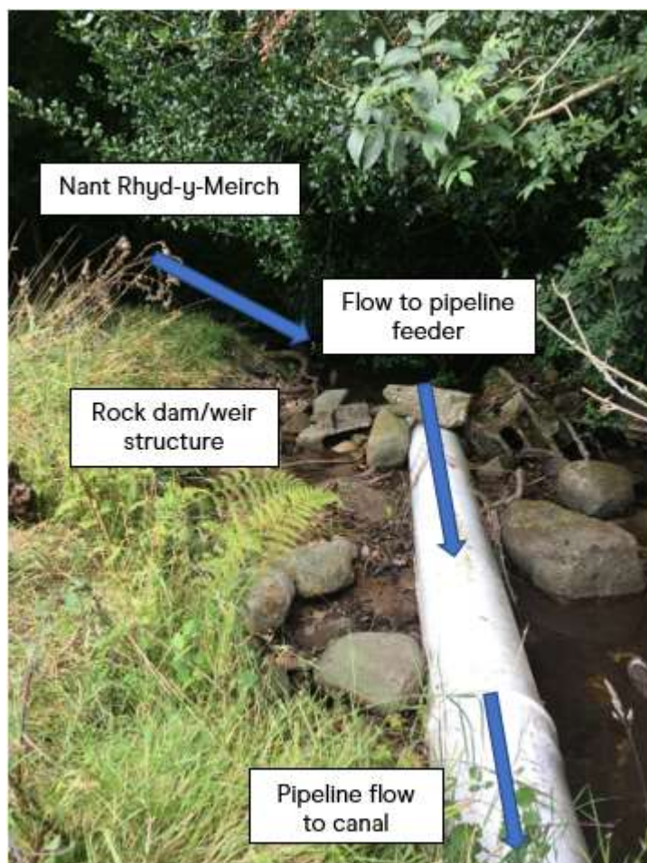
Photo 4: Pipeline to canal, downstream of abstraction point A 17.08.11
