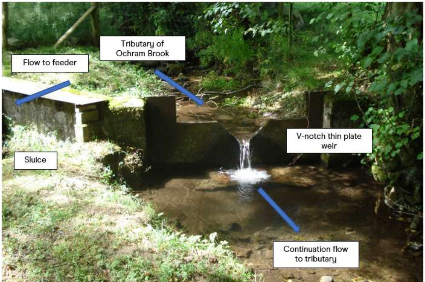
Photo 4: Sluice, settling chamber and V-notch weir: flow to canal 17.08.11
