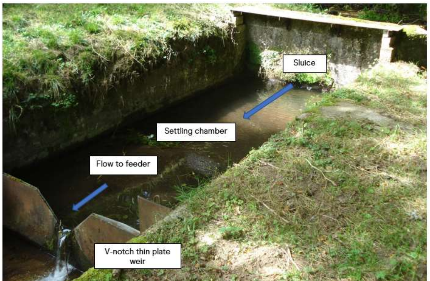
Photo 4: Sluice, settling chamber and V-notch weir: flow to canal 17.08.11
