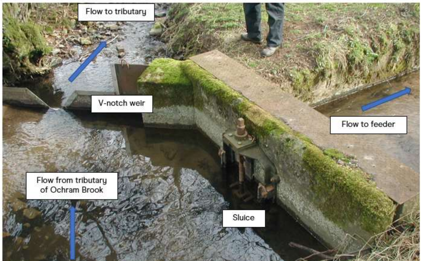
Photo 2: Sluice to feeder channel and continuation flow to tributary, looking downstream
