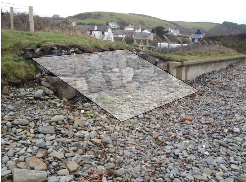
Figure 3: ramped excavation - constructed to access the lower area.
