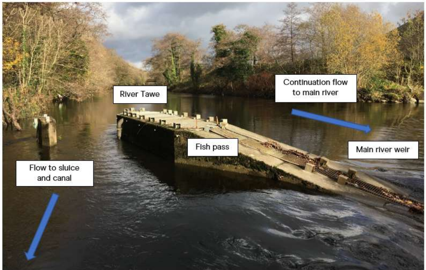
Photo 2: Main river weir with fish pass and downstream continuation flow 13.11.18
