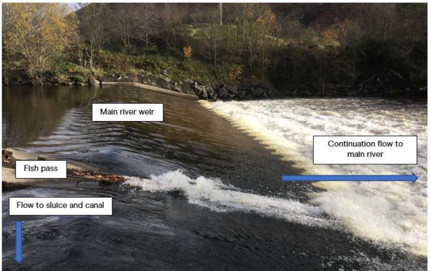
Photo 2: Main river weir with fish pass and downstream continuation flow 13.11.18
