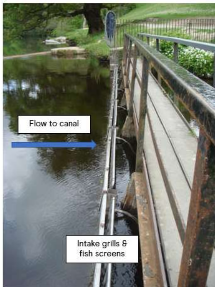
Photo 3: Abstraction at Llantysilio Feeder – intake grilles and fish screens 02.08.13
