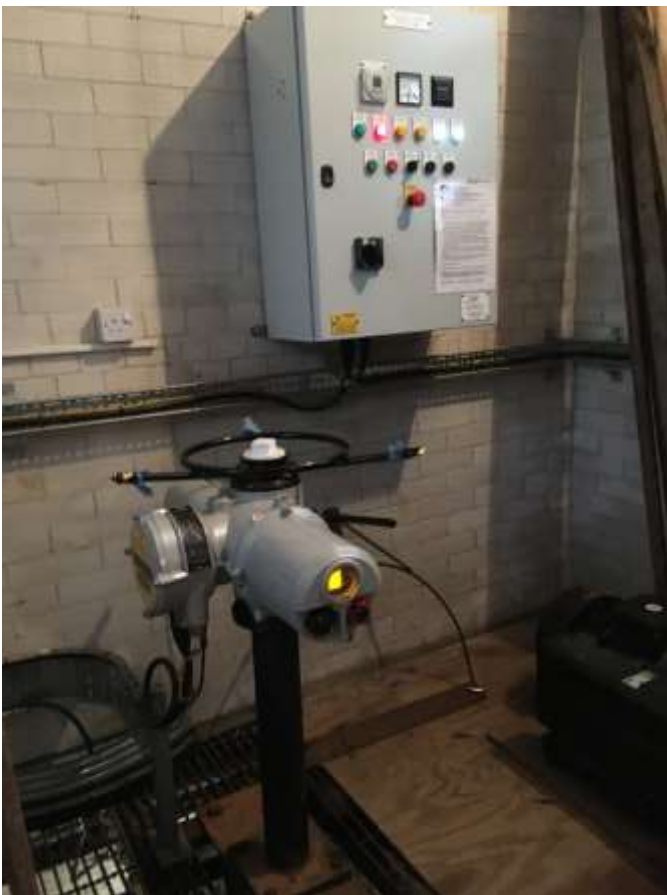
Photo 6: Downstream sluice controls inside Meter House 29.01.19
