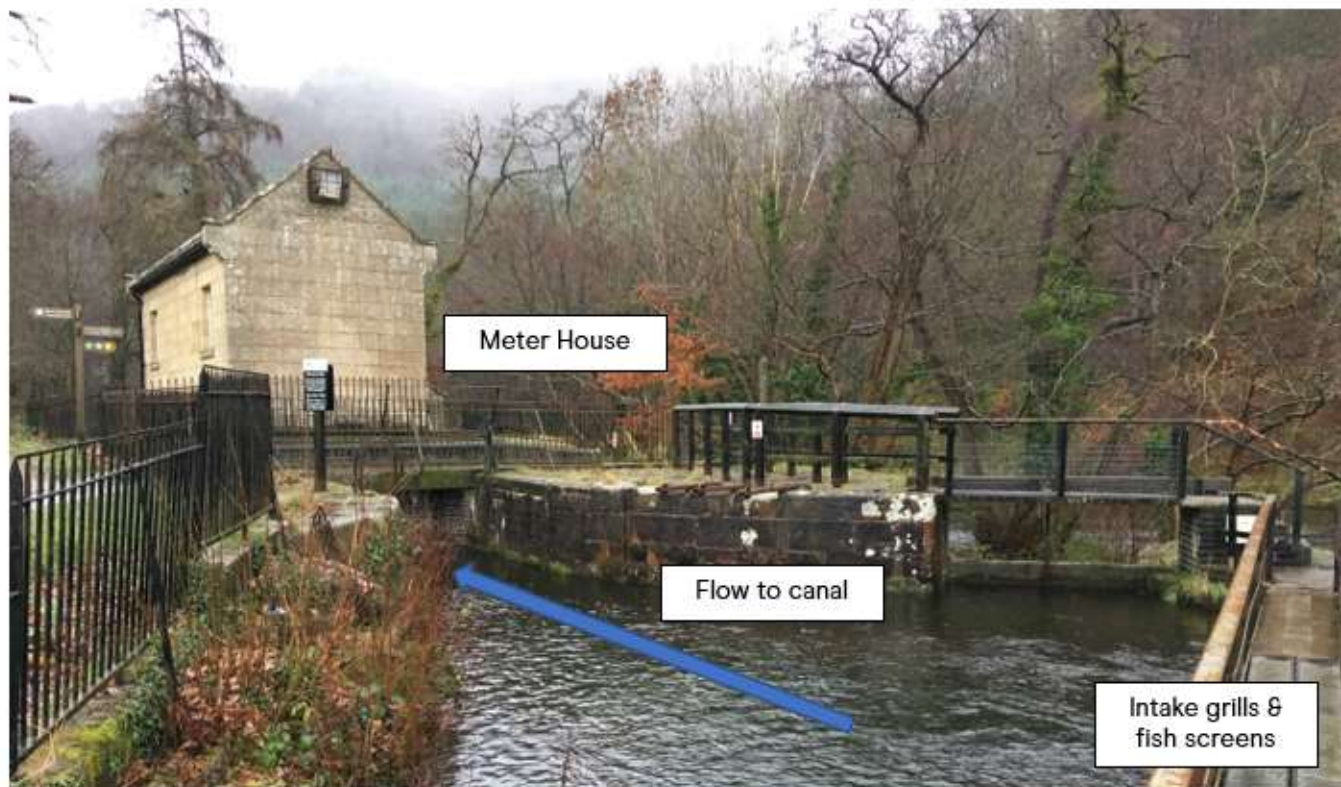
Photo 4: Flow to the canal downstream of grilles & fish screens and Meter House 29.01.19
