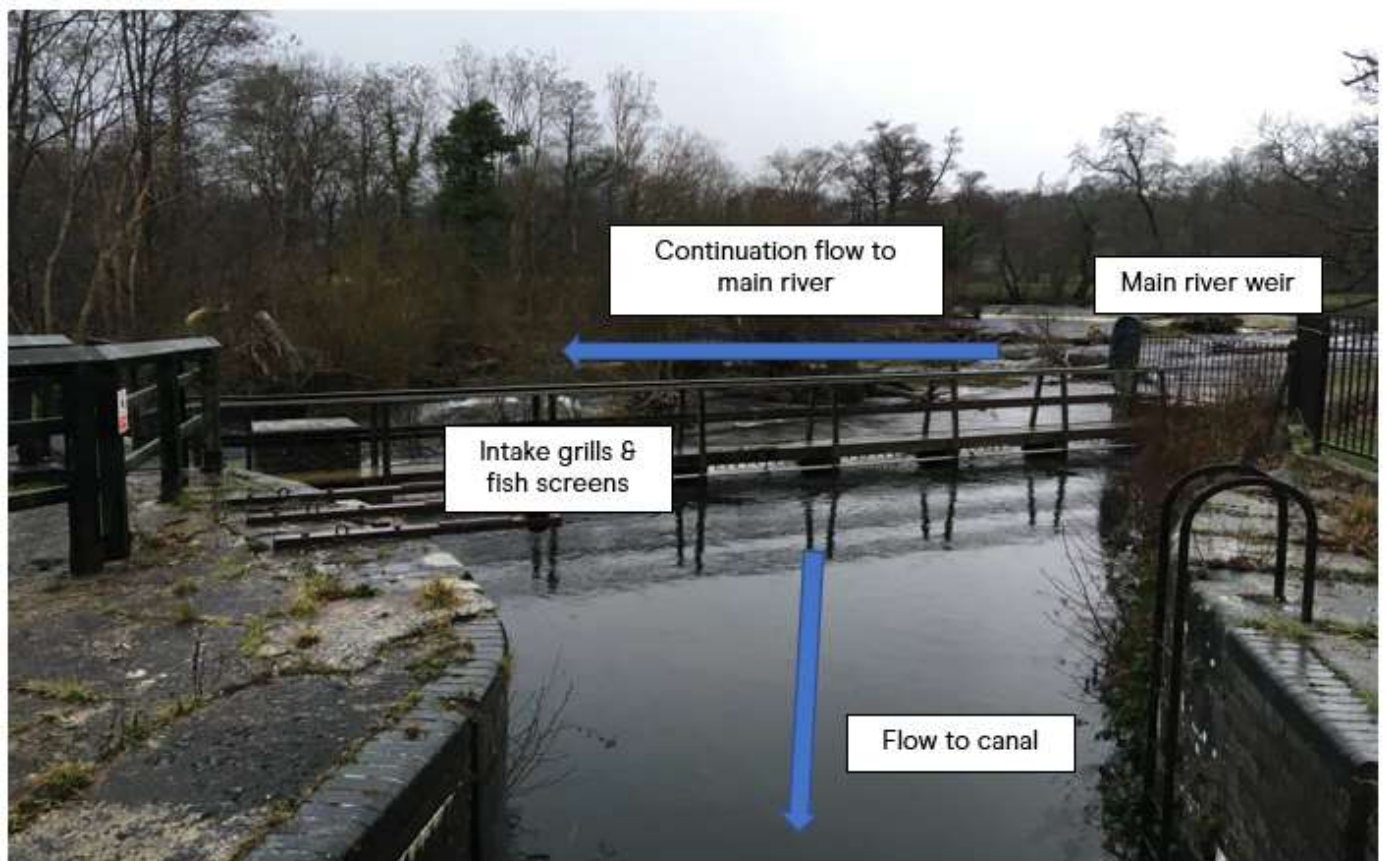
Photo 2: Horseshoe Falls with intake grilles & fish screens 29.01.19
