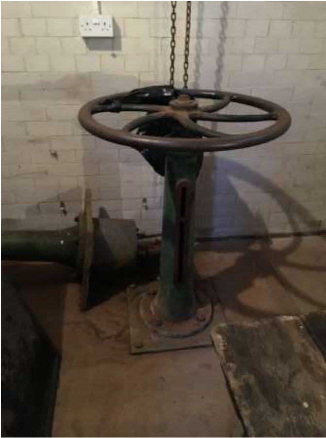
Photo 5: Upstream sluice controls inside Meter House 29.01.19
