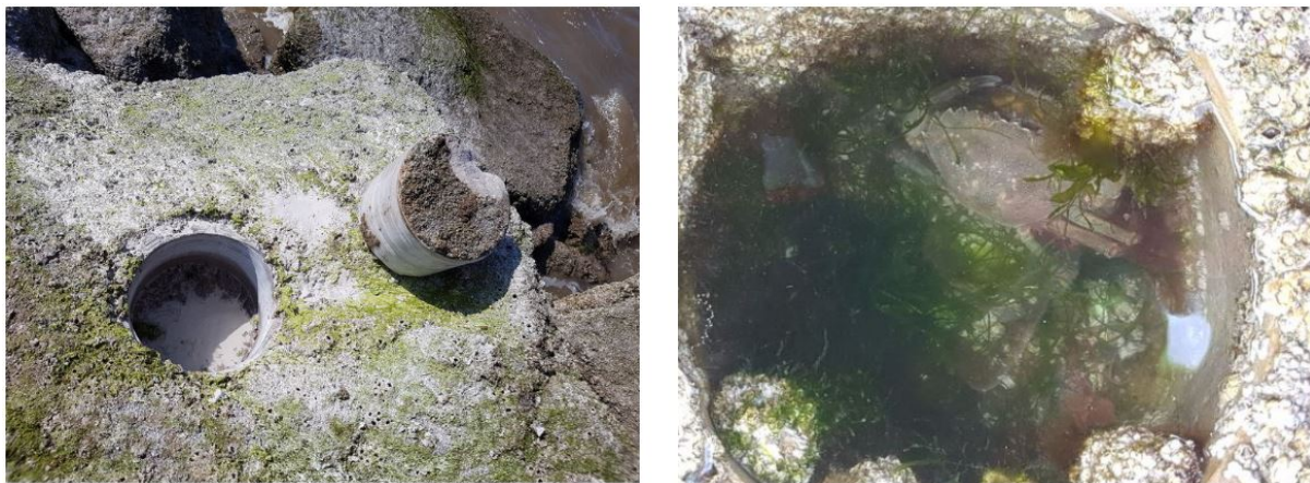
Image 4. Examples of core-drilled granite for biodiversity enhancement by Aberystwyth University
