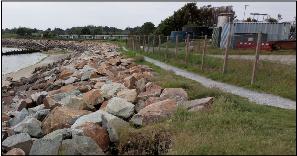
Image 1. Previous sewage treatment plant (STP) that has been demolished and existing revetment that will be redesigned and realigned
