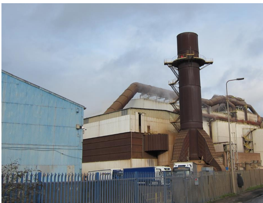
Photograph 2-1: Stack A1 (furnace fume extraction)
