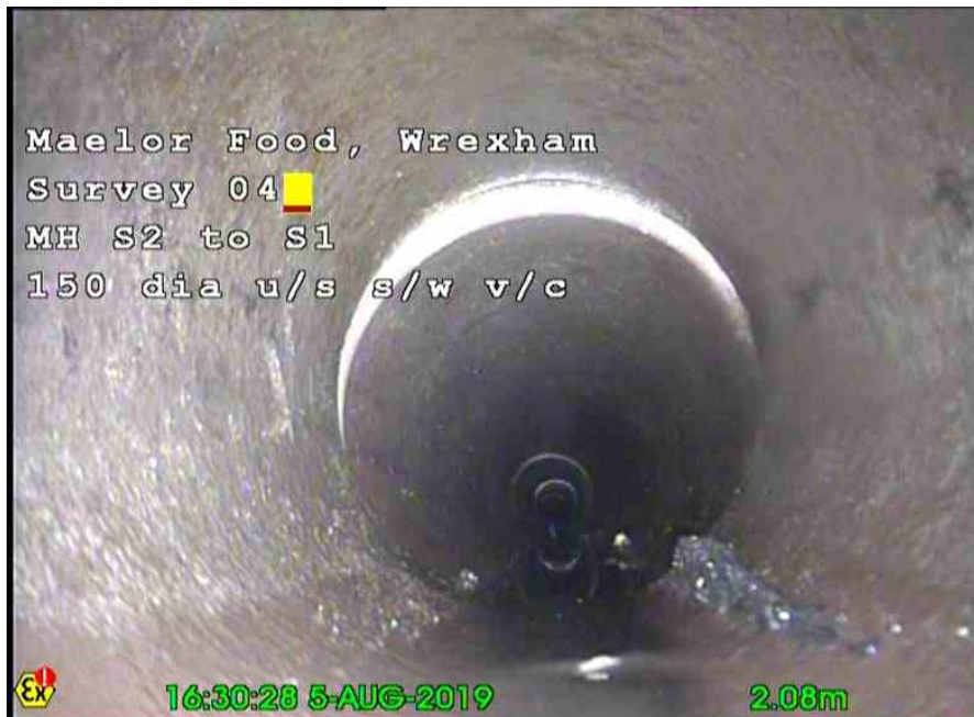
S1X_89ad0789-a15f-4878-9a5f-28bd63b423fc_20190831_152209_383.jpg, , 1.99m Joint displaced, medium
