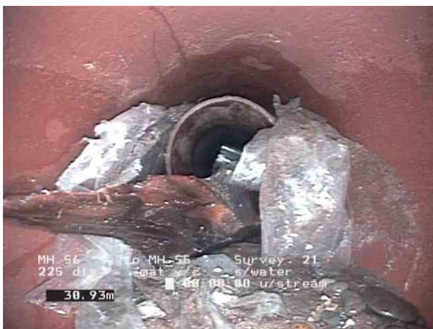
S5X_b9a80b22-8a74-4485-8e98-95494038ba3a_20190831_154920_610.jpg, 30.93m Obstacles built into structure from 3 o'clock to 8 o'clock, 40% cross-sectional area loss
