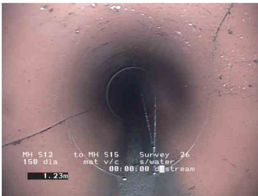
S12X_50c434ec-2dba-482b-9d2c-ca77962d7113_20190831_155227_638.jpg, , 1.23m Fracture, circumferential from 1 o'clock to 9 o'clock
