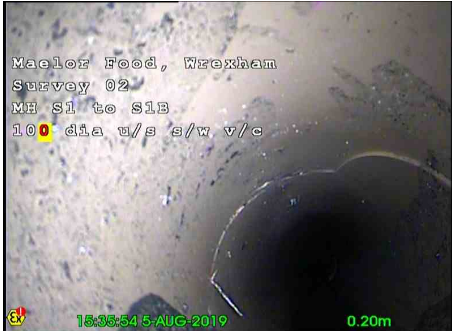
S1BX_b156a5fb-e561-4582-bede-1cc2464815b3_20190831_151707_263.jpg, ,0.50m Fracture, circumferential from 8 o'clock to 11 o'clock
