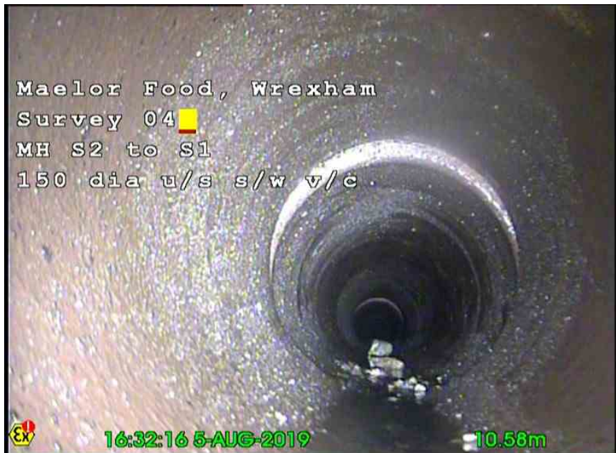
S1X_c2a9191b-cc80-48d4-ba1f-9bb299068c05_20190831_152321_169.jpg, , 10.58m Joint displaced, medium
