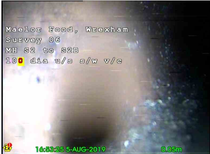
S2BX_dc71426f-fe8d-45e7-95a7-78c20e875e39_20190831_152700_651.jpg, , 6.50m Settled deposits, coarse, 90% cross-sectional area loss
