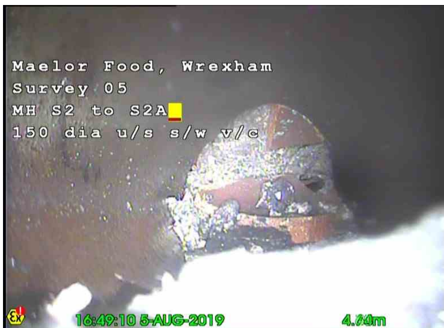
S2AX_bfa92ef3-b481-4bc5-9f70-bad4e8cc225d_20190831_152534_770.jpg, 4.75m Collapsed drain or sewer
