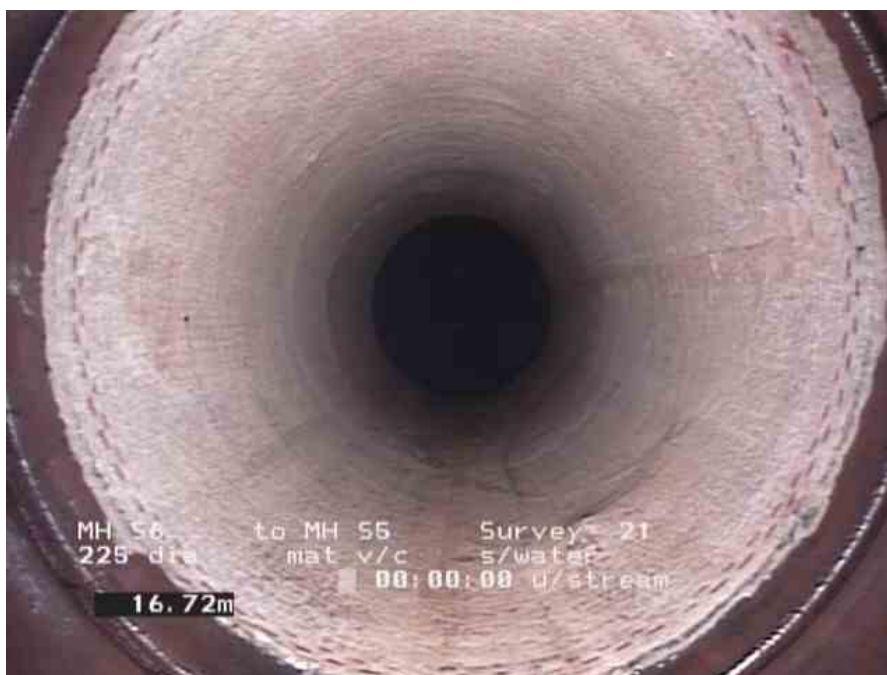
S5X_07b4e33c-280a-48a8-8a40-a63b7ba0fc5b_20190831_154800_512.jpg, 16.72m Point repair, localised lining from 12 o'clock to 11 o'clock
