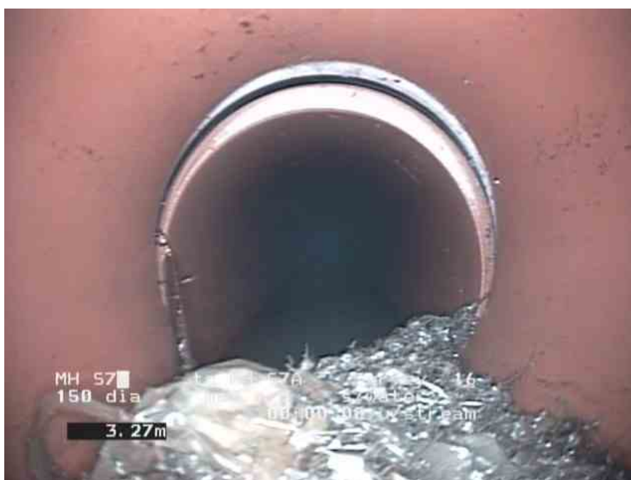
S7AX_ca0b25ba-d372-4765-bb6d-46a92d997eda_20190831_154342_689.jpg, ,3.27m Joint displaced, medium
