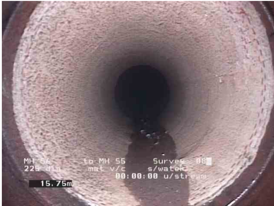
S5X_49f79797-b73d-4239-8ce6-aa7553c7f003_20190831_152956_167.jpg, , 15.75m Point repair, localised lining from 12 o'clock to 11 o'clock
