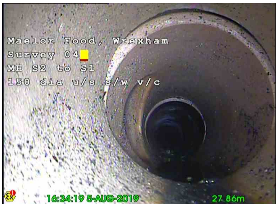
S1X_57513bce-5eb0-43a4-871b-4ff319134bec_20190831_152428_691.jpg, , 27.83m Joint displaced, medium
