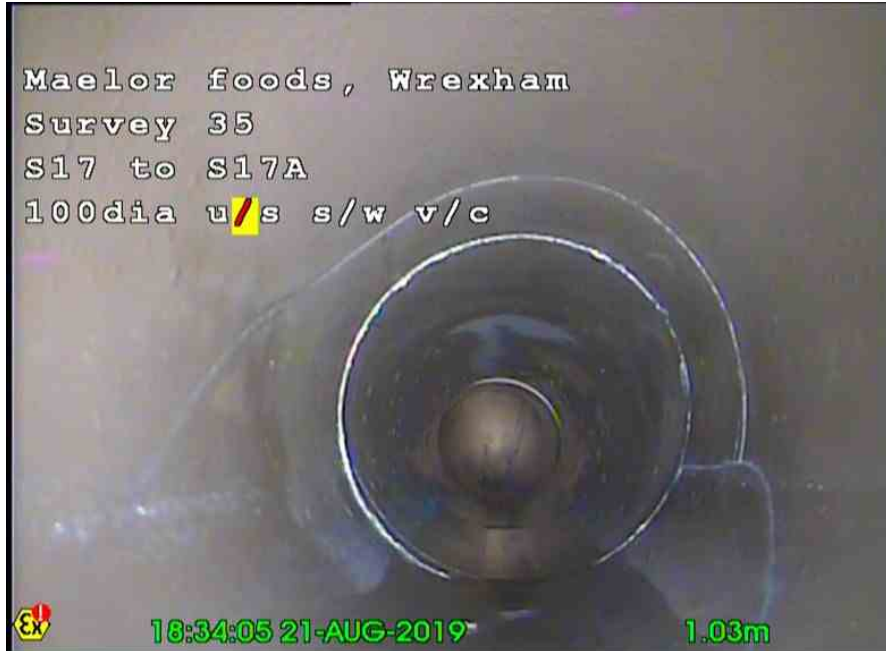
S17AX_3af38ca9-55df-4d11-aa63-5b291ee504bf_20190901_143608_665.jpg, 1.02m Fracture, circumferential from 8 o'clock to 4 o'clock
