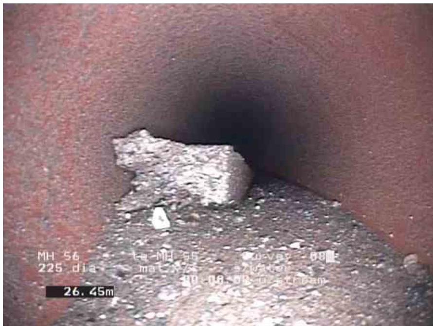
S5X_8b46bbdc-0edf-4bba-bda0-e6bca71cf85c_20190831_153057_297.jpg, , 26.45m Settled deposits, fine, 50% cross-sectional area loss
