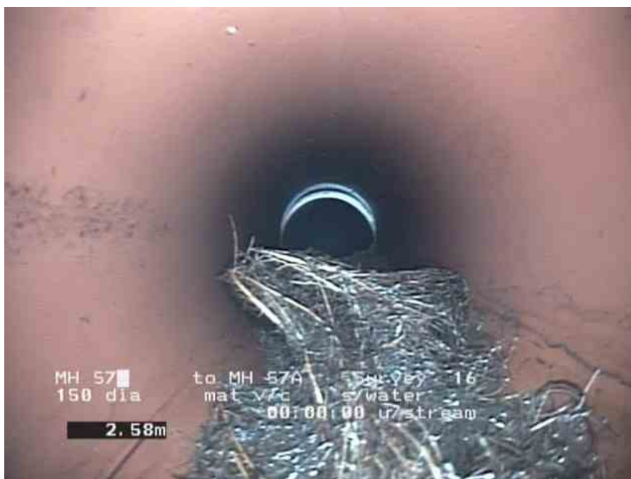
S7AX_4e6393c3-12bd-4b5e-a1d9-61dbb4d7ea56_20190831_154328_075.jpg, ,2.66m Roots, mass, 40% cross-sectional area loss
