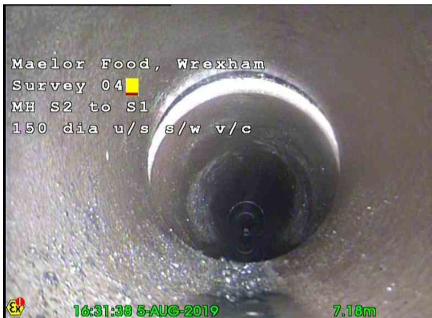
S1X_f076290c-a229-4d32-9721-ffcd157d96cf_20190831_152254_213.jpg, , 7.18m Joint displaced, medium
