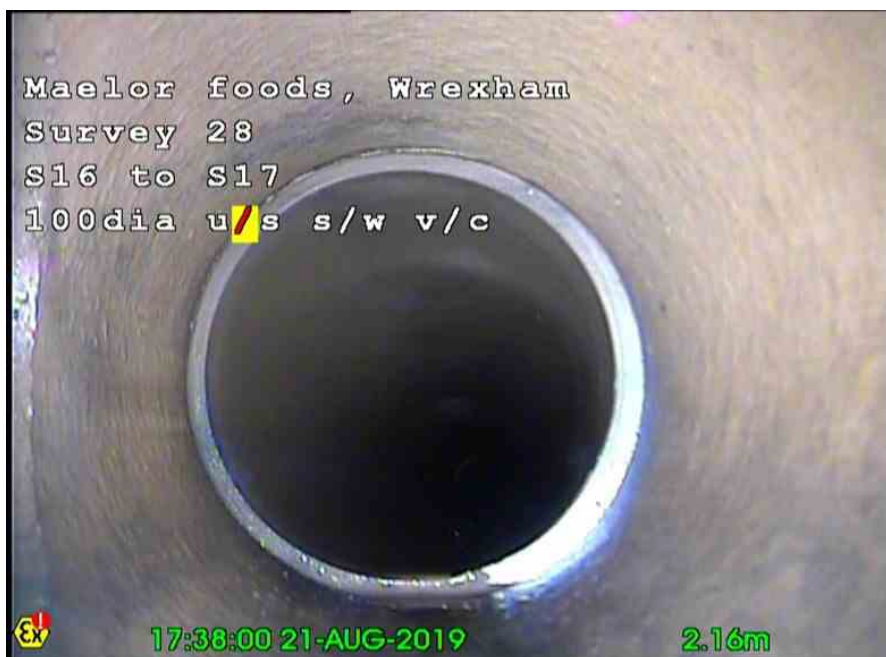
S17X_61dff4ed-df79-473d-bb73-f6807787cc87_20190901_142902_769.jpg, , 2.16m Joint displaced, medium
