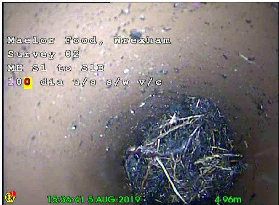
S1BX_2ba055a9-13eb-4fbb-90e1-8ddb62a9c48_20190831_151739_040.jpg, ,4.84m Roots, mass, 80% cross-sectional area loss
