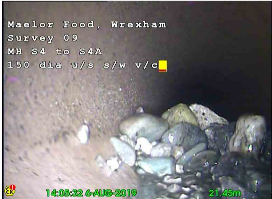
S4AX_cf6e278b-8b76-4949-9463-6e8631fc79dd_20190831_153519_168.jpg, , 21.54m Settled deposits, coarse, 30% cross-sectional area loss
