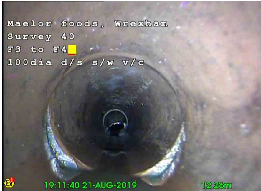
F3X_6abd29a4-a382-4ec8-91d1-ca435f9bd642_20190901_144154_920.jpg, , 12.35m Joint displaced, medium
