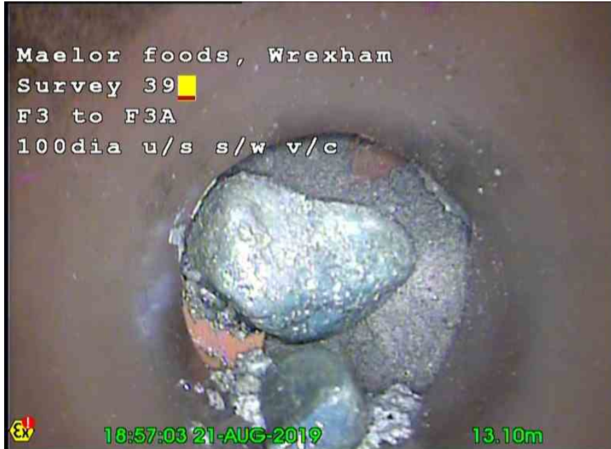
F3AX_08d98c01-fe34-4350-b699-8c7494d63b9b_20190901_144049_496.jpg, , 13.10m Obstacles, brick or masonry in invert from 12 o'clock to 11 o'clock, 95% cross-sectional area loss
