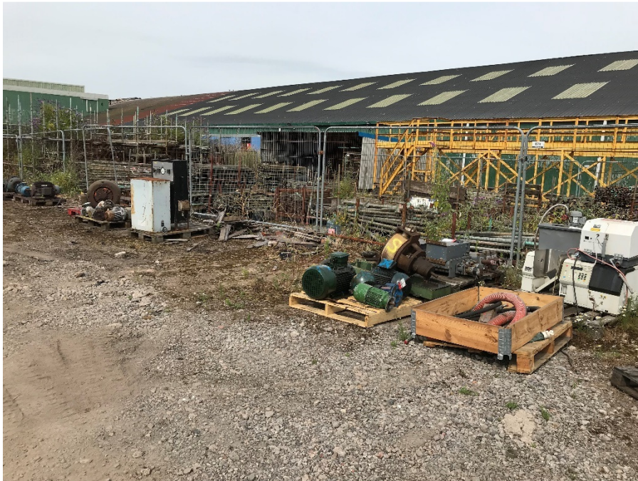
Scrap / spares storage on bare ground
