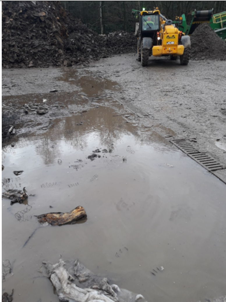
Photo Three – Contaminated water entering drainage gully.
