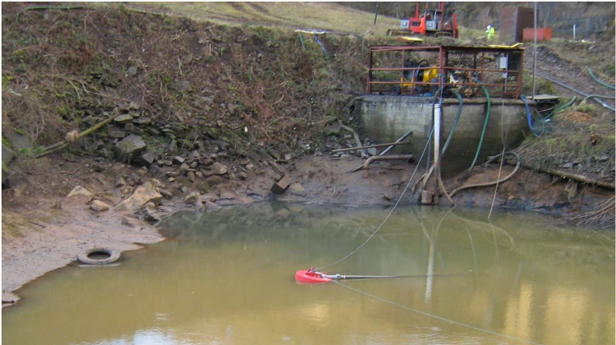
Photograph 1 – the float switch pump following installation in the sump in 2010
