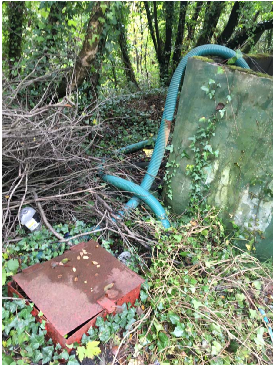
Photograph 5 – pipework from the sump towards the disused tank with meter housing (red box)
