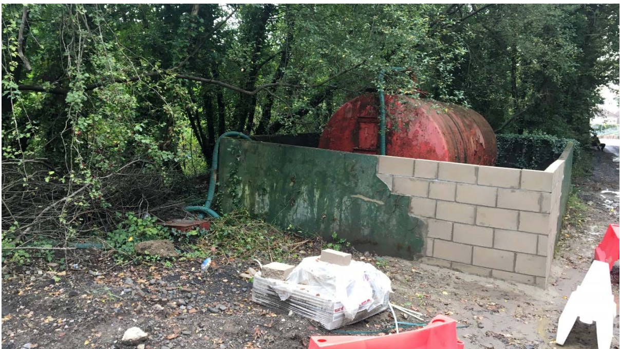
Photograph 4 – pipework from the sump towards the disused tank (water is then diverted to sewer or Cwmrhydyceirw Stream)
