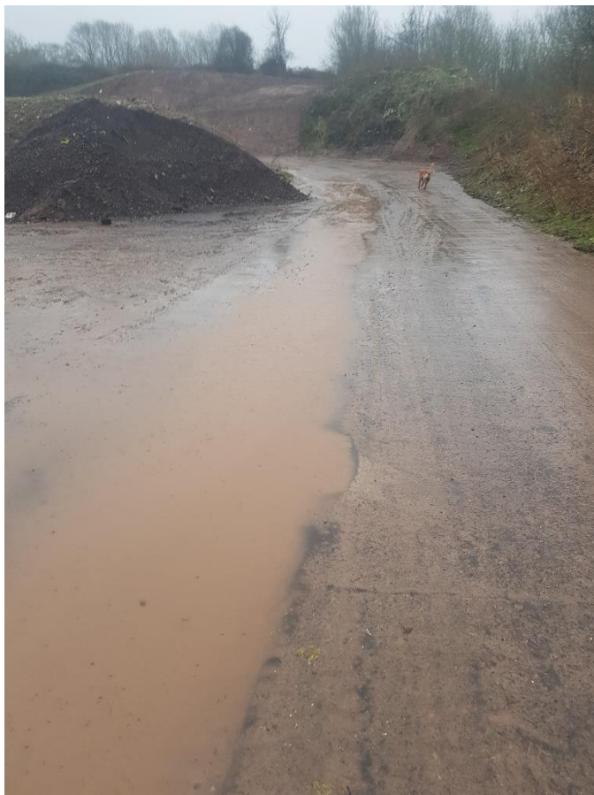
Runoff flowing along slab across southern section of site.
