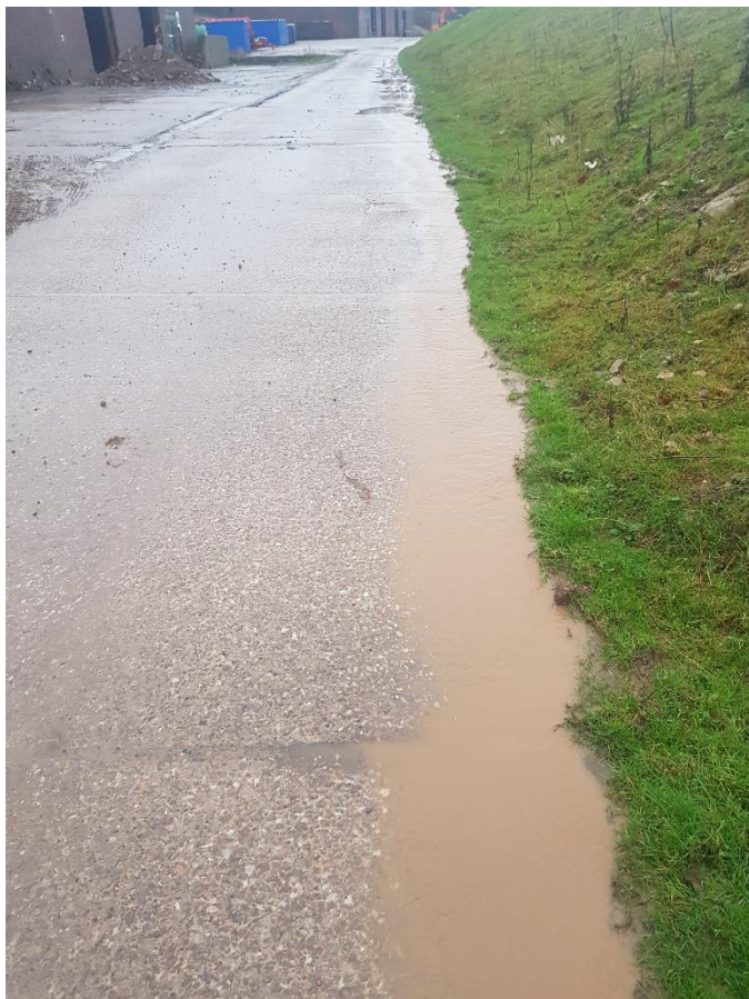
Runoff flowing along soils on the edge of the slab. Not clear if kerbs have been removed or buried.
