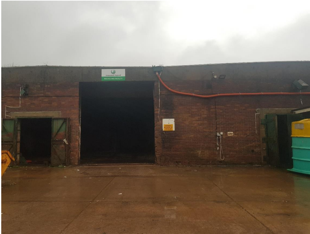
Building 1 – Southern elevation with flexible pipe taking runoff from the roof to a soakaway to the east of the building.
