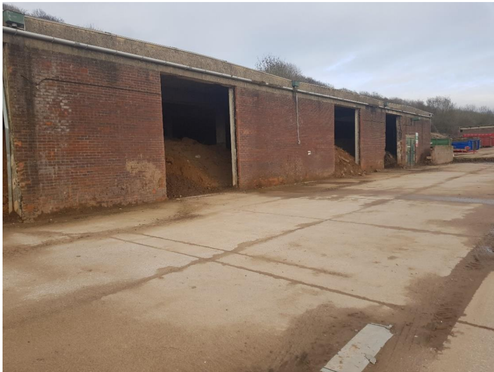
Building 4 – Guttering along front of building, collecting rainfall from valleys between bays.
