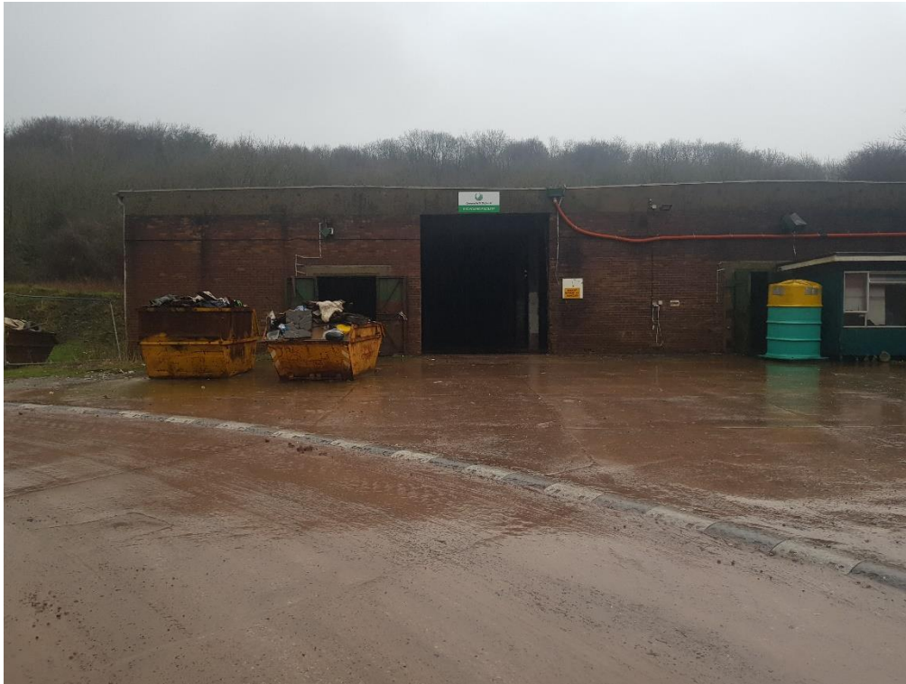
Building 1 – Southern elevation, bund across forecourt to contain and direct runoff from the forecourt into a 1200l tank.
