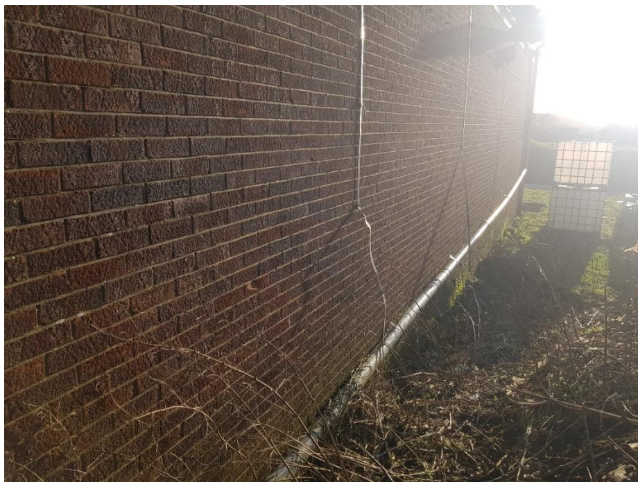
Building 4 – Rainfall from guttering at front of building being channelled to vegetated areas behind building.
