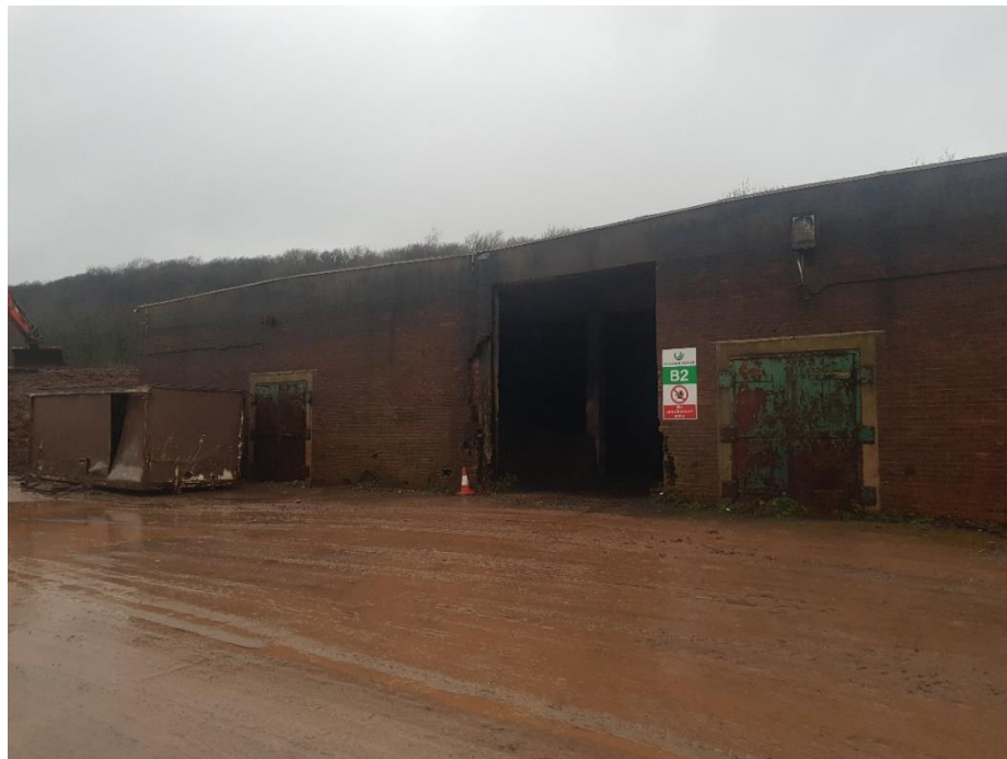
Building 2 – western section – Damage to brickwork around vehicular door. Brickwork is not structural as the doorway is supported by a concrete portal frame.
