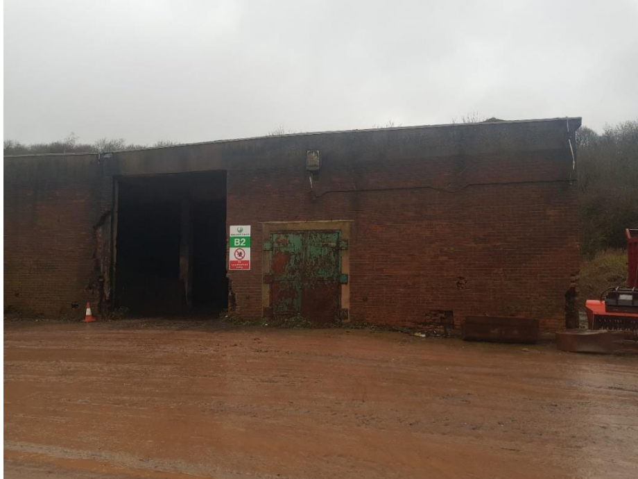
Building 2 – Southern elevation with 3.5m wide vehicle access door and pedestrian door.
