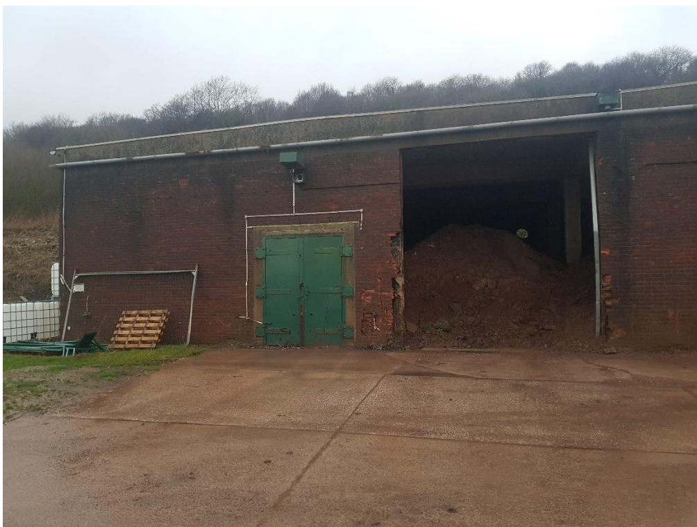
Building 4 – Western side – Further damage to brickwork around vehicular door.
