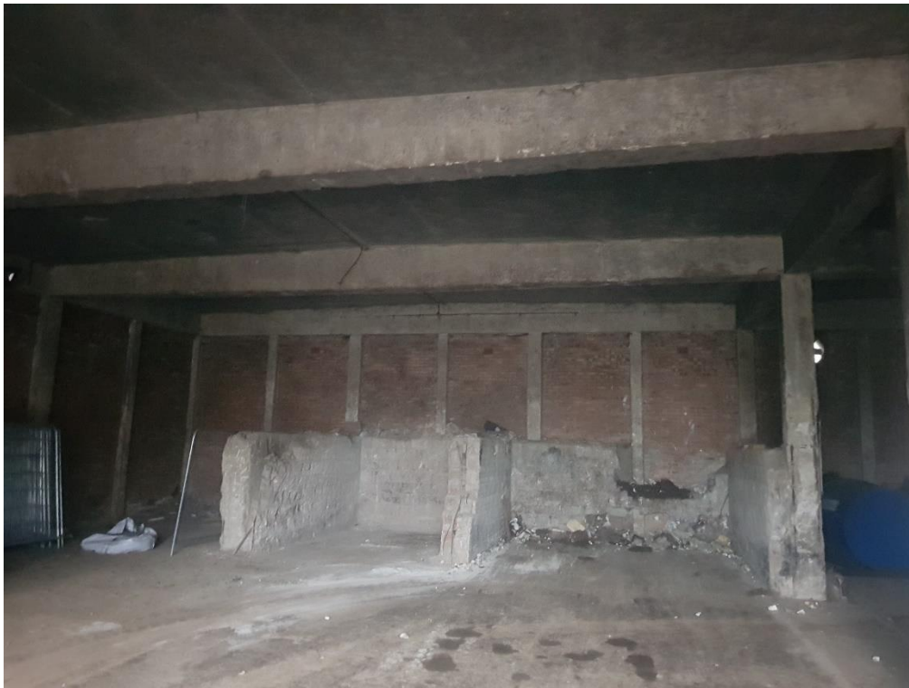
Building 1 – Quarantine bays and brick infills between concrete pillars making up the walls.
