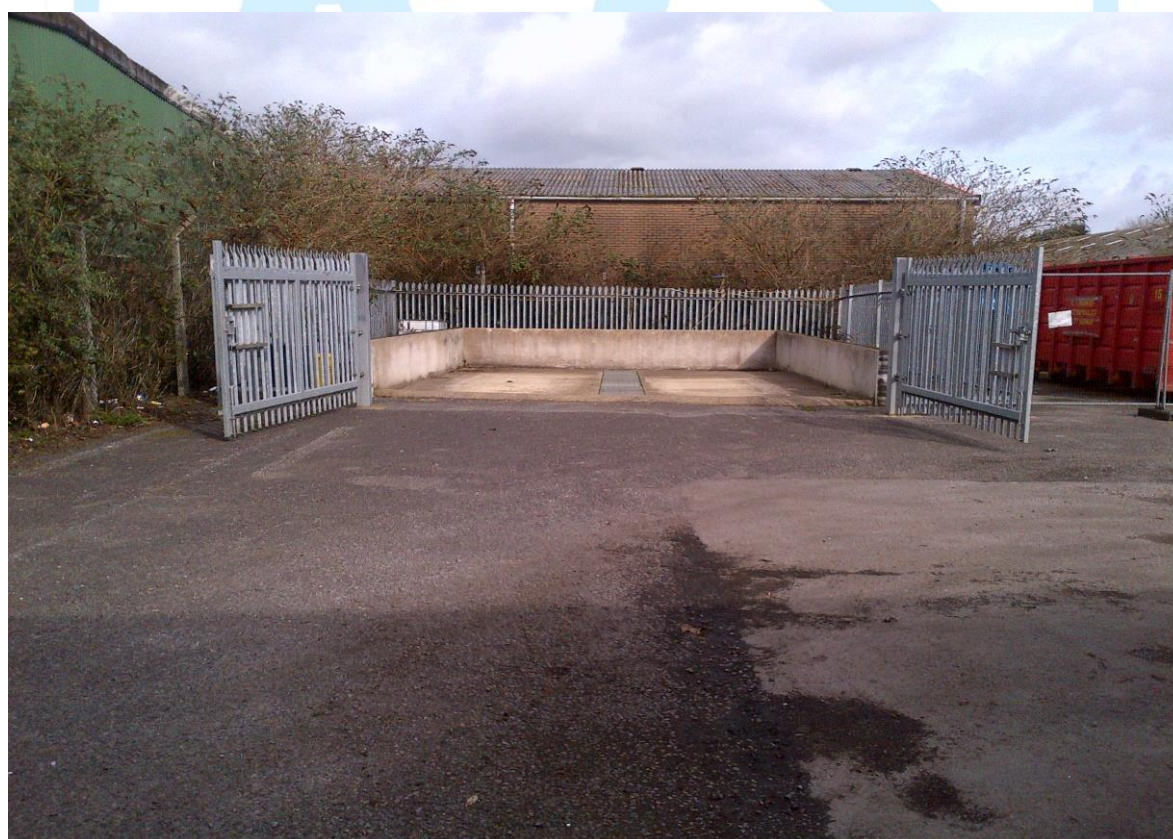
General view above of the WTS (Waste Transfer Station) with the gates open
